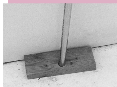
Small blocks of pressure-treated wood, drilled with deep holes the diameter of the pipe, support uprights and protect the deck.
