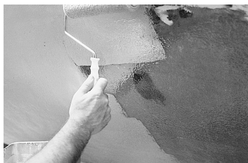
Interprotect 2000 is rolled over a smooth, fair hull surface.
