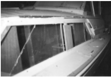
Removing windows and fitting mahogany corners.
