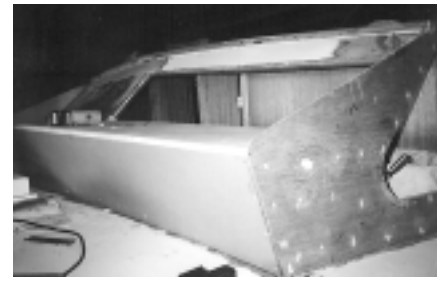
Forward seat takes shape. Only half of the window opening has been filled in with plywood.
