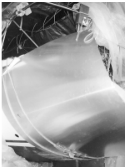
(top) Line drawn across at top apex forms contour of one-off aluminum mold. Plasticine fillet fills the gap at the transom and makes a smooth, curved joint for glassing; (bottom) Wedges and cardboard shims inserted under lines close-fit the mold against the hull.
