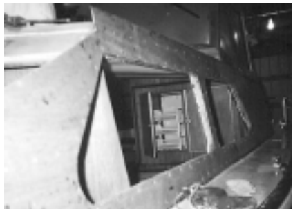
Lauan underlay glued to the sides to blend in the new construction.
