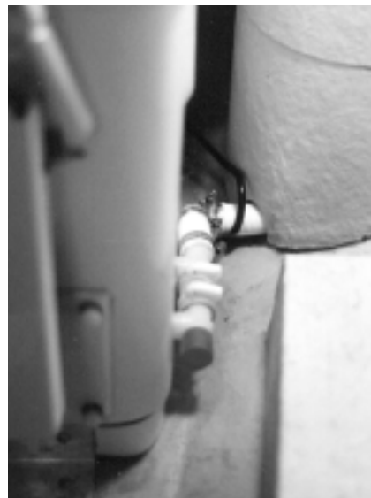
Overflow hose for excess liquids connects to a holding tank.
