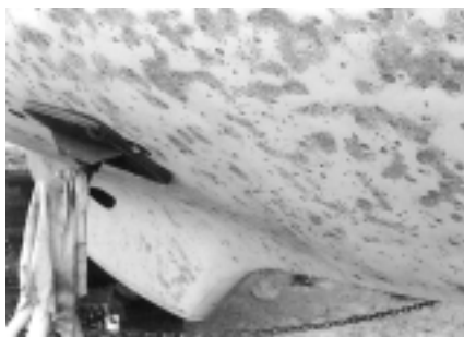
After sandblasting, the extent of Princess II 's blistering became obvious.
