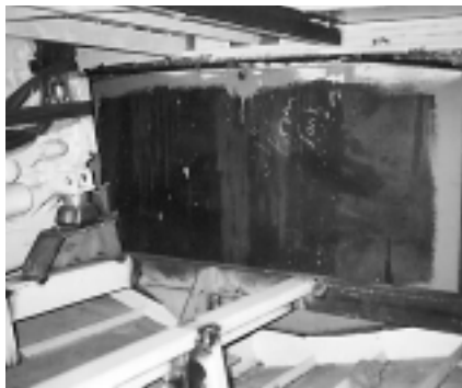
For diesel only, sheet steel, spec ASTM-A93 in 14-gauge, is a lower-cost alternative to stainless steel, but not as long-lived.
