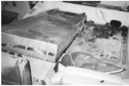
Crevice corrosion on the surface of these aluminum gasoline fuel tanks caused by poor installation.
