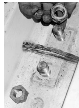
Typical top-end installation with backing plate and washer.
