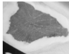
Whitish cracks radiating outwards indicate damaged laminate. Grind the laminate to remove all delaminated glass and reinforce laminate.
