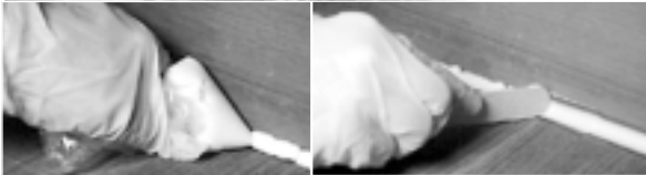
New longitudinal and athwartship floor supports coated with unthickened epoxy resin for moisture protection, then epoxy
