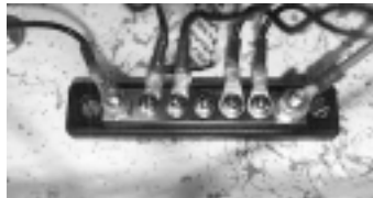
Dedicated terminal block for negative wires.
