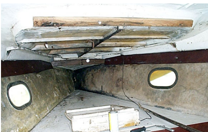
A previous owner had "improved" the original design by raising the foredeck several inches, supporting the underside with a web of wooden stringers attached with polyester resin. The result was a cracked and leaking deck, rotten deck ply and stringers. Holes were epoxy filled, epoxy fillets reinforced the stringers and the entire overhead was coated with unthickened epoxy.
