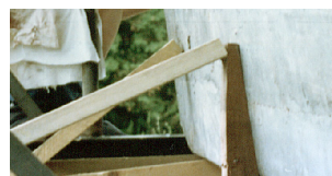
Framework of wooden braces and cleats supports the cut off piece.
