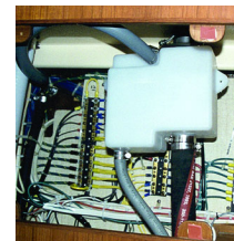
Completed installation of Splash-Stop. A more compact, redesigned Vetus Splash-Stop is now available.
