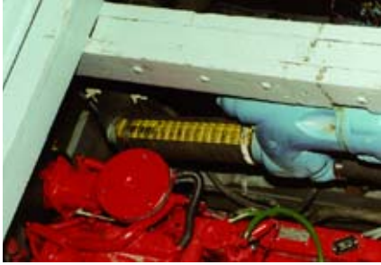
Hoses were replaced with certified ones, including a certified Vetus exhaust hose.
