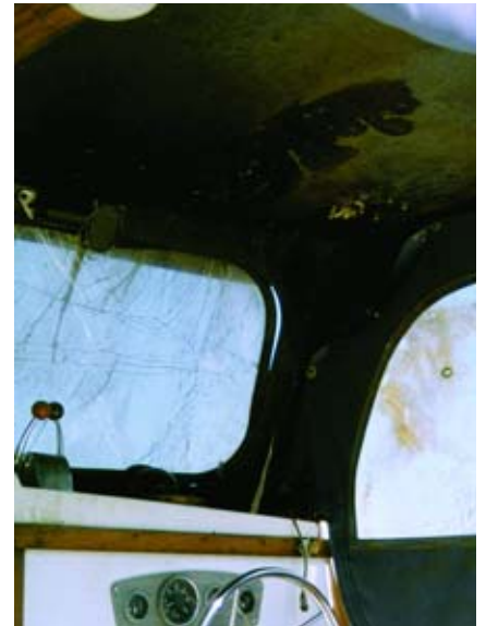
When lightning struck the VHF antenna on this 8m (26') Grover cuddy cabin while cruising Chesapeake Bay near Annapolis, Maryland, it burned a hole through the cabintop, and the resulting shockwave shattered the windshield. Note the hole in the hardtop and the burn pattern on the left above the helm. Owner Morgan Wells and two other men in the cockpit were injured. The boat did not have a lightning protection system.
