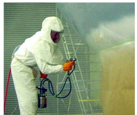
Spray application of the white boot stripe begins with a light tack coat and may need three to five coats to cover. Yellow and other bright colors take even more coats.
