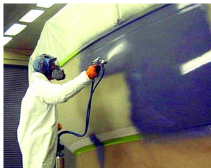
Primer spray application, at least two coats are needed.
