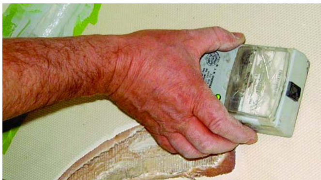
A high moisture reading signifies that water has entered the deck core.
