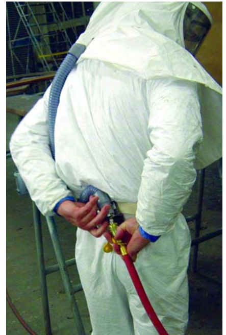
Spraying highly toxic two-part polyurethane paint requires protective gear including a fresh-air supply to the technician. Disposable suit is made of vapor-proof Tyvec.
