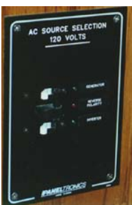
FIGURE 9 SAMPLE AC SELECTOR PANEL.
