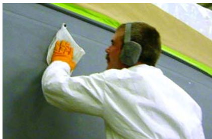
Final dust removal with a tack rag.
