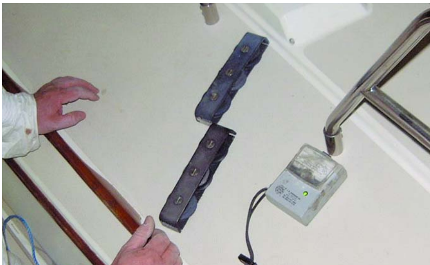
Examine deck fittings regularly with a moisture meter and rebed any that give a high moisture level to prevent further damage.
