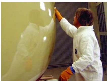
Professional painter, Earl Hadcock, makes repairs and completes masking. He uses the recommended solvent wash to clean the hull and remove any wax or oily residue that may cause paint adhesion problems later.
