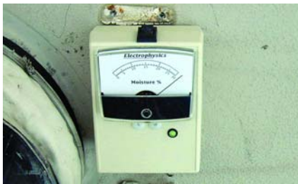
Pegged moisture meter identifies delaminated area.
