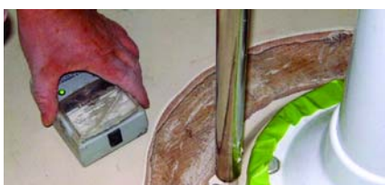
Moisture check shows drying in progress.
