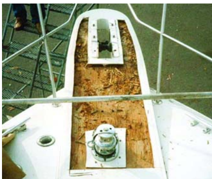
Digging out the bad core
