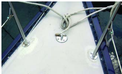
Another common problem area is a bow pulpit base before repair.
