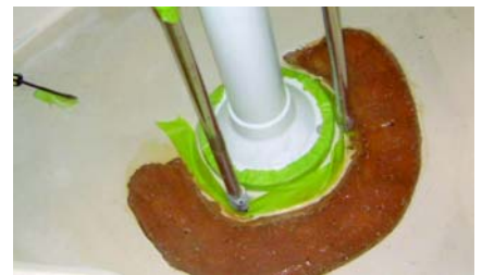
Core replaced with solid glass filler ("potted").
