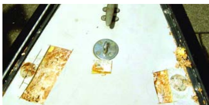
Removal of wet balsa core at the pulpit bases.
