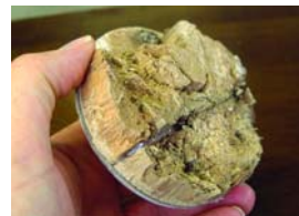
A "coupon" removed with deck laminate still attached.
