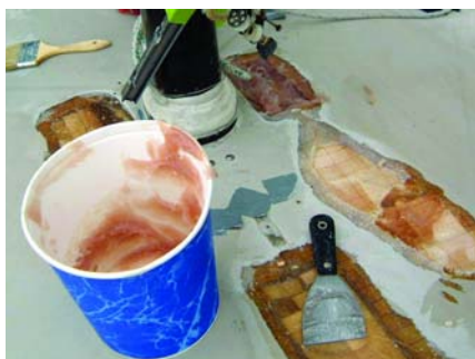
Potting of new core underway. Note chopped mix in bucket ready to be troweled into place.
