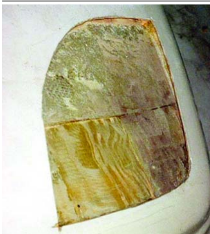
Damp core that is intact is not removed but left to dry.
