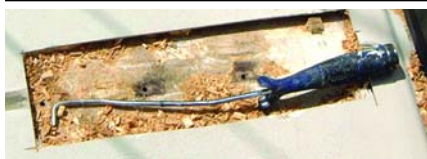
Removing core under the babystay track utilizes a customized tool for digging core out from under the upper laminate.
