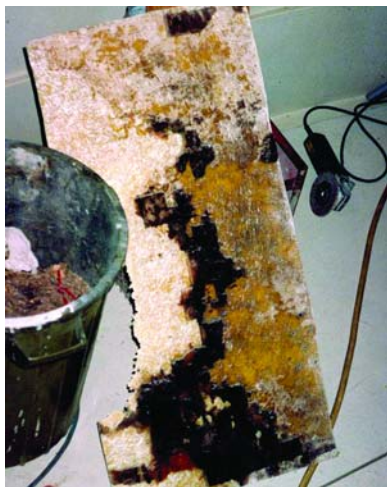
A partially rotted balsa core sample.
