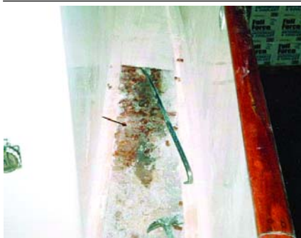
Bad core exposed.
