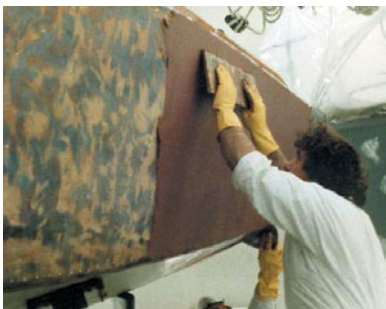
Leveling or "screeding" filler with a piece of scrap Plexiglas. Also touch ups with a small 10cm (4") putty knife.
