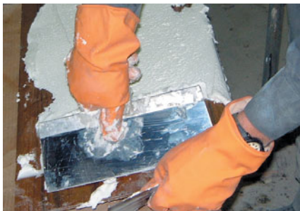
(left) Working the fairing compound to get even consistency. (right) Coarse filler is mixed to a peanut-butter consistency for applying to vertical surfaces.
