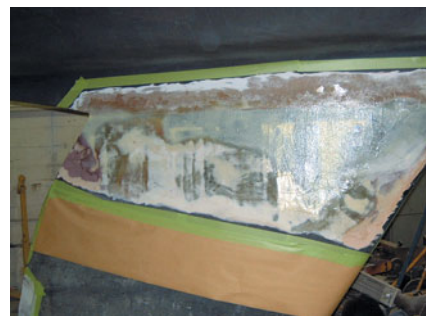
Keel repair after two fills.
