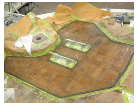
Deck repair ready for sanding and filling.
