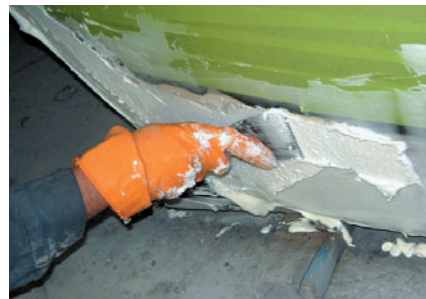
(left) Working the fairing compound to get even consistency. (right) Coarse filler is mixed to a peanut-butter consistency for applying to vertical surfaces.
