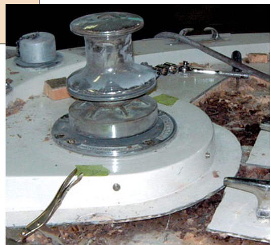
Delamination caused by improperly caulked windlass fasteners and hawsepipe hole results in a costly foredeck repair.
