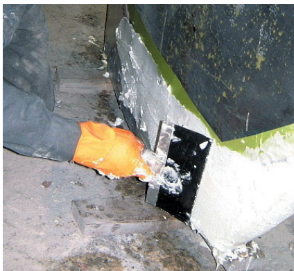
"Screeding" is physically easier and less time consuming than sanding.
