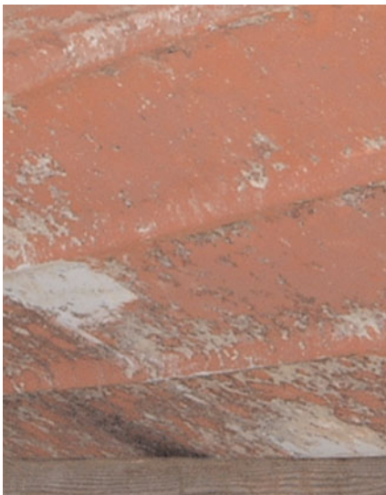
Old worn-out paint should be stripped before recoating.
