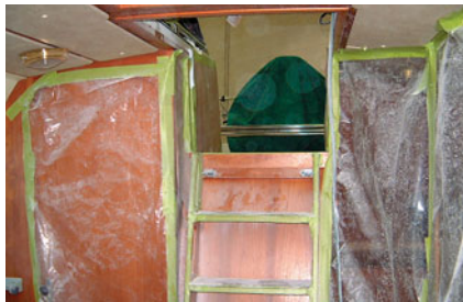
Grinding fiberglass inside requires protecting the interior with a dust barrier of plastic sheets.
