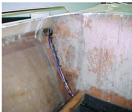
Wires should be tied and secured. A very neat job!
