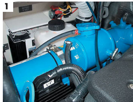
1 Typical heat exchanger located on the top of an engine usually towards the back. Cap is used to fill and maintain the system.
