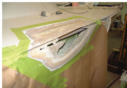
C&C 25: After prep grinding, the repair is ready for new glass lay-up. Note beveled edge, which represents a scarf ratio ranging from 8:1 to 12:1 for this 6mm (1/4") thick hull.
