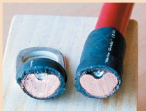
Example of what a good crimp looks like after the hammer blows. Note how the strands of the wire and the walls of the lug appear as solid copper.
