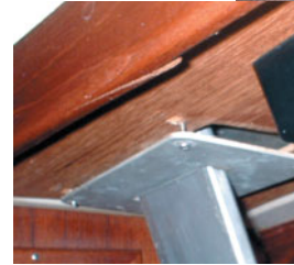
right) Dufour 38 was not as lucky. Note broken mahogany inner liner and cracked glass headliner. (bottom) C&C 35 suffered shifted shelving, bulkheads and broken interior trim.
