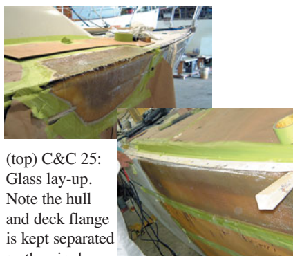
(top) C&C 25: Glass lay-up. Note the hull and deck flange is kept separated so the vinyl rubrail can be reinserted. (bottom) Dufour 38: Note new PVC core just visible through the new laminate. (top) C&C 27: Large overlap around location of original hole dictated by extensive stress cracking.
