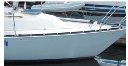
C&C 25: After painting, launch rerigging. Hull still needs a final buff to blend in the edges of the repair.
