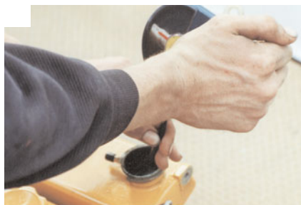
Remove the filler cap on the heat exchanger and use an antifreeze tester to check the strength of the coolant. Change coolant as needed, depending on storage temperatures.
