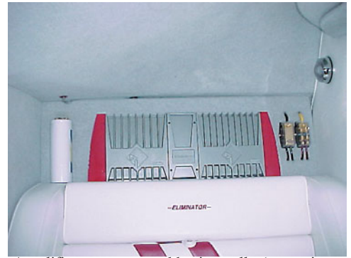
Amplifiers are mounted horizontally (or vertically) in an area that is dry and well ventilated. A capacitor (shown on the left) assures that the amps get continuous power. Fuses appear at right.
