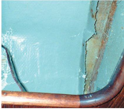
C&C 35: Broken tabbing in a hanging locker.
