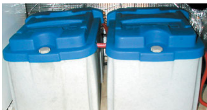
Screw-down covers that hold these batteries securely in place, even in rough seas. They also cover the terminals so nothing metallic can short-circuit them.
