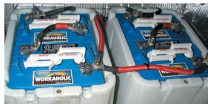
This boat needs to be protected against acid spilling from the battery. A drip tray might help but a battery box is better. Note how these boxes attach to the boat by external screws. Never drill holes through the bottom of the boxes to fasten them down as this gives any leaking acid a path to leak from the container.
