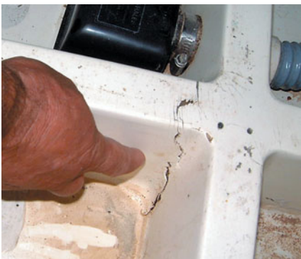
(top) This sub-floor grid suffered fractures during a 3-knot grounding on a rock. (bottom) Close up of cracked grid.
