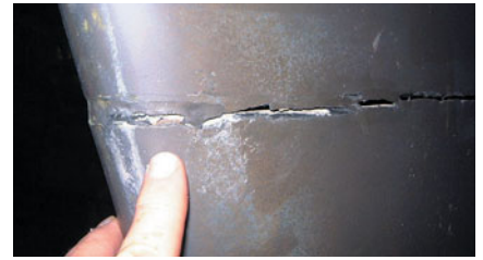
A separation this wide at the keel-hull joint indicates the keel needs to be dropped and rebedded.
