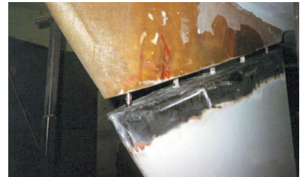
The keel-hull joint is cleaned and prepped for reinstallation with new sealant and chocking epoxy.
