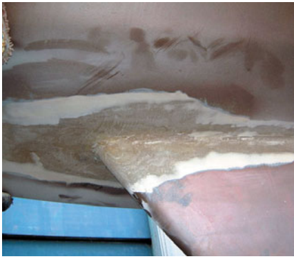
Several small core samples (note circular marks) are taken to guide the removal of delaminated sections of the floor grid.
