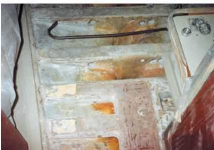
During repairs the mast step and keel stub structure needed reinforcing beyond the original scantling to restore the original structural integrity.
