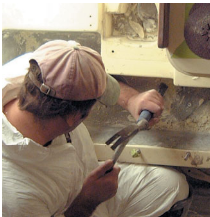
Removing broken secondary bonds in tight spots requires a hammer and chisel.
