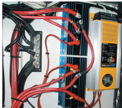
Smart chargers and battery isolation diodes allow the alternators to charge multiple batteries.
