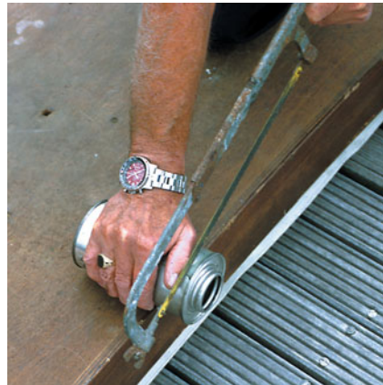
The pipe was removed and the filter unit taken out onto the dock where the casing was cut off leaving just the base and threaded spigot.
