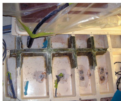
(top) Delaminated floor pan has been ground away leaving the structural grid ready to be re-glassed to the hull. (bottom) Floor grid in early stages of new glass lay-up.
