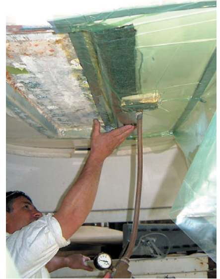
A vacuum bag makes overhead work easier and gives superior glass-to-resin ratios.
