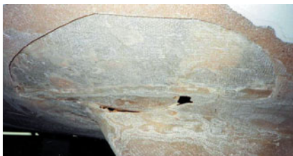
"She's a hurtin' unit." Wet and delaminated core must be removed and replaced.
