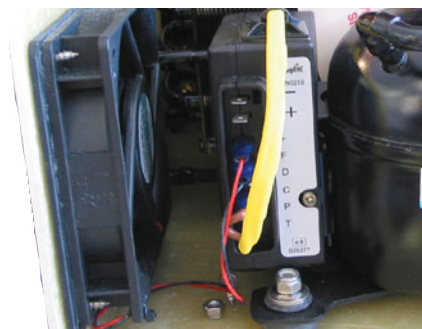
(top) Keep condenser grill or radiator free of dirt and dust. (bottom) When a fan fails, shown on the left in this photo, replace it with a readily available computer box fan.
