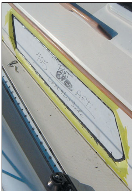
Masking for perimeter caulking.
