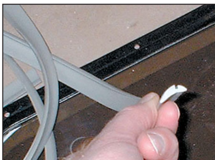
(left) Rubber gasket is pushed in until detent locks in frame. (right) Detent in sealing gasket.
