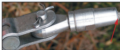
(top) Water seeping under the wire has caused this swaged stainless-steel terminal to pit and crack. (bottom) Waterproof the wire terminal joint with a dab of silicone sealant.
