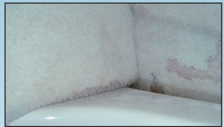
Water leaks at portlights have traveled to wet the headliner as seen by the unattractive staining.
