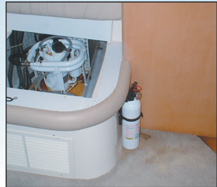
The air-conditioner compressor condensate collection pan didn’t drain properly and trapped water overflowed and soaked the carpet (under the fire extinguisher). Boat owner was unable to determine the source of the water.
