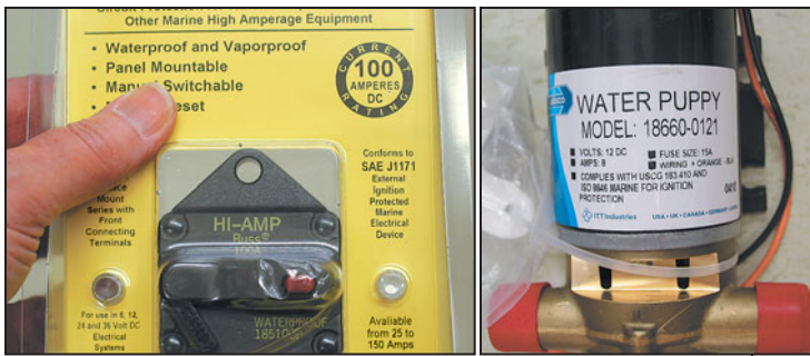
(left) This high amperage circuit breaker is ignition protected as it conforms to SAE J1171. (right) This water pump's label states that it complies with USCG and International Standards Organization (ISO) regulations for marine ignition protection. (bottom) The manufacturer's label says this marine water heater is ignition protected. Information on the specific testing criteria met will likely be found in the accompanying owner's manual.
