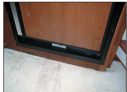
Condensate drain for this refrigerator was plugged and water had been leaking onto to plywood cabin sole beneath carpet. Flooring and plywood subfloor have both delaminated.
