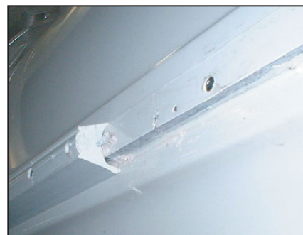
Shoebox style hull-to-deck joint on a Searay 480. Solid PVC rubrail overlaps joint.
