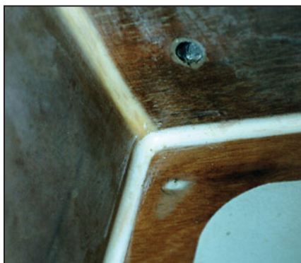
A fillet fills the gap between the joint, strengthening the bond at the joint and supporting the secondary bonds. To form, apply a thick paste of epoxy resin and spread with tongue depressor.
