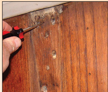
Leaking chainplates are a common problem. Look for telltale dark stains.
