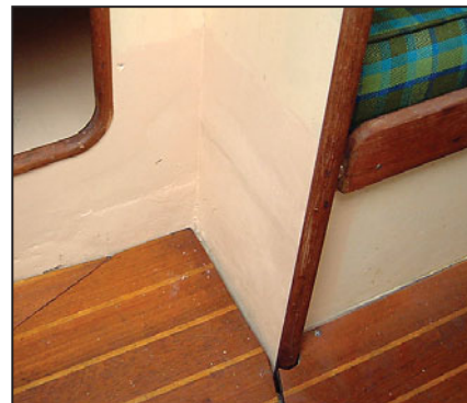
Finished bulkhead repair after tabbing with a glass overlay applied to the butt joint and painted.
