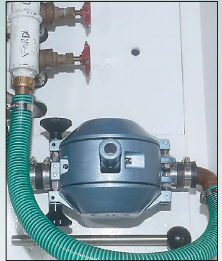
If the pump is leak free, reattach the mounting brackets and piping. Clip the operating handle neatly into position next to the pump ready for use. This job took about four hours, excluding filling and painting the pump housing.
