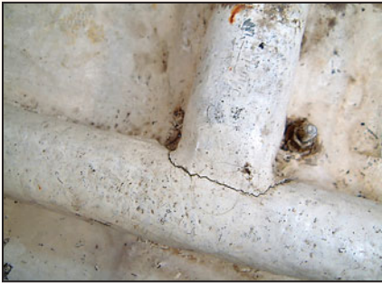
(top) The left hand stringer here was overloaded by a grounding incident and has broken just forward of the mast step (the mast step has been removed). (bottom) Closeup of cracked rib and stringer joint.
