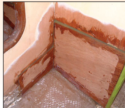
Ongoing bulkhead repair ready for tabbing. Note butt joints ready for glass overlay.
