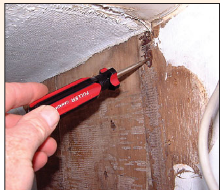
Check for rot with a sharp probe.
