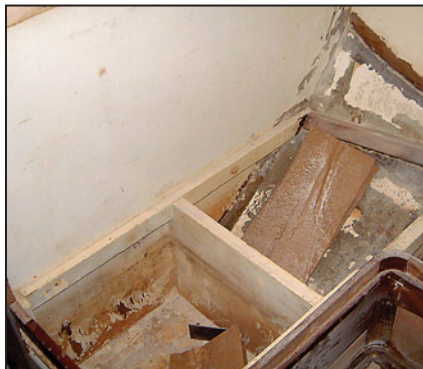
Bulkhead deterioration begins in damp poorly ventilated areas.
