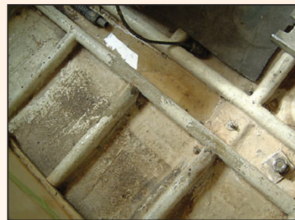
Example of the structural grid system below the cabin floor of a 33' (10m) sailboat. Note the two parallel stringers running fore-and-aft adjoining the athwartship ribs. (Refer to photos of damage and repair throughout this article.)
