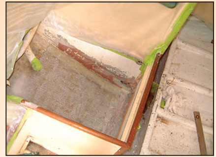
Delaminated tabbing at the base of this main bulkhead has been removed with a grinder. Note plastic sheets for dust protection.
