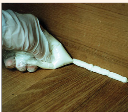
New bulkhead piece in place and ready for filleting. Gap at bottom has been packed with thickened resin.
