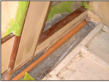
Dry fitting a new wood stringer core on the sailboat stringer shown on page 19.
