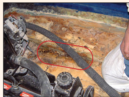
The dark area is where wet floatation foam has contributed to rotting the aft stringers under the cockpit floor of a 24" (7.3m) sterndrive-powered cruiser. The wet foam and rotted plywood stringer both require replacement. (See photo of repair under "Glass Lay-up.")
