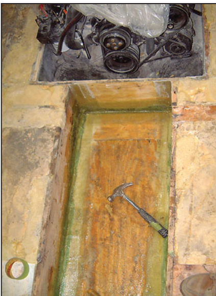
Location of the fillet and overlapping layout of typical encapsulating glass secondary bonds.
