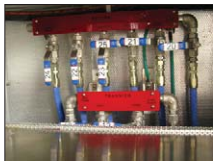
Best is to have all valves organized in a logical manifold system.
