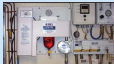
Algae-X FPS fuel-polishing system is an affordable solution to eliminate water, sediments and particulate while reconditioning and stabilizing the fuel.
