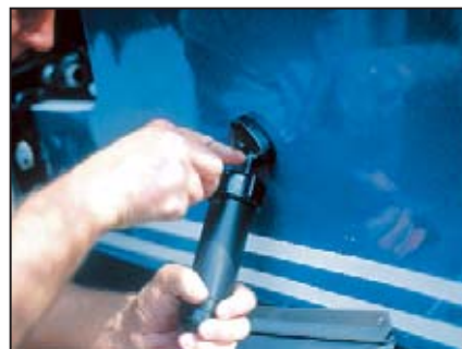
After applying a generous bead of caulking around drilled holes, actuator is fastened to the transom.
