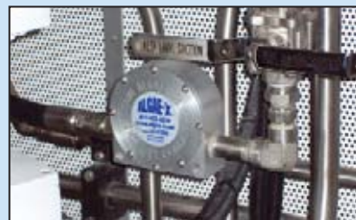
Algae-X utilizes magnetic fuel conditioning technology to enhance engine reliability and prevent engine damage.
