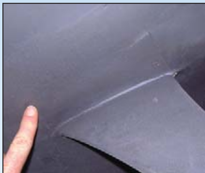
This strut is not glassed in yet is very similar to the one shown in Figure 3. The recessed flange has been filled over and faired smooth and hairline cracks trace the outline of the flange. The thru-bolts are buried just under the filler.
