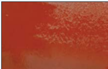
Surface contamination caused an orange peel effect on this surface coated with Toplac, a one-part polyurethane paint.
