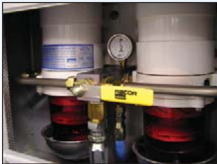
Dual-mounted water separating filters. Note vacuum gauge.
