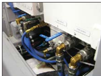
Clearly labeled valves.
