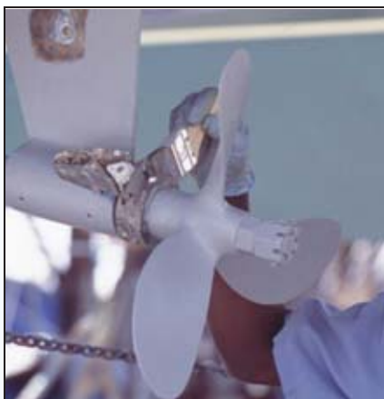
Final coat of Interprotect 2000E applied to running gear.
