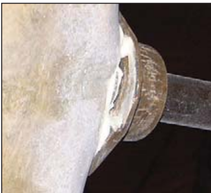
This small opening at the side of a stern tube bearing is an inlet for cooling water. It should never be blocked with caulking or antifouling.
