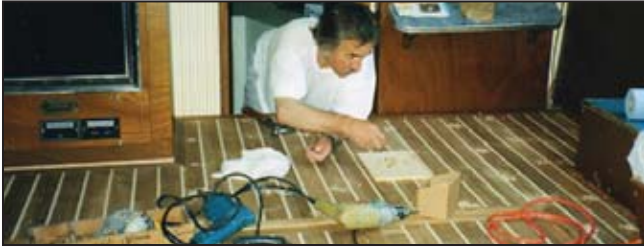
All screw heads are covered with teak plugs. Note that the holly strips align properly with adjoining panels.
