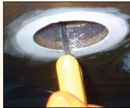
After removing core, the gap between the skins is grouted with chopped fiber and resin.
