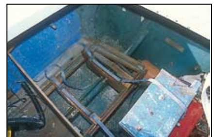
Strap kit fastened to custom mounting beds ready to install the heater.
