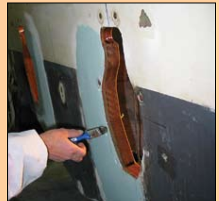
Epoxy resin was brushed on to seal exposed wood around cutout.
