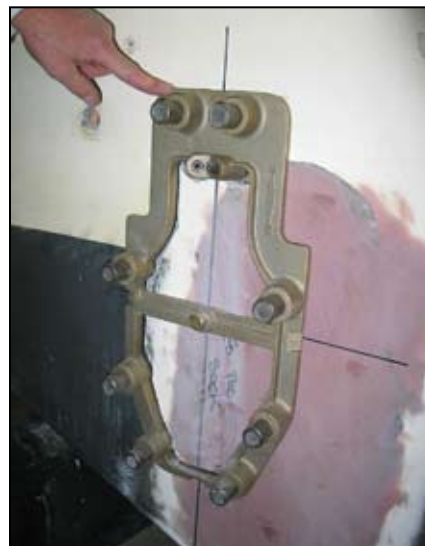
Installing transom cut out fixture.
