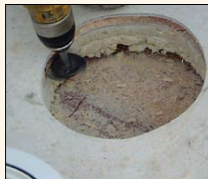
To prepare to pot a fitting remove the core with a rotary cutting tool.
