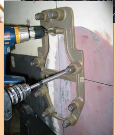
Transom assembly matched to "X" dimensions and the fastener holes drilled.
