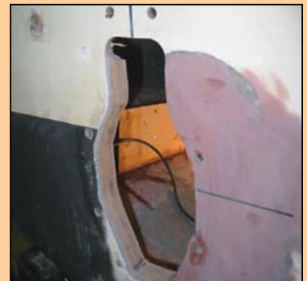
Mercury transom cutout fixture, part number 91-55852A2, was used to maintain tight tolerances that will eliminate water leaks.
