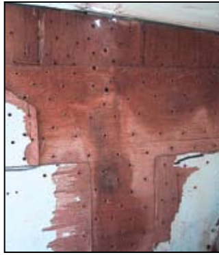
Series of holes drilled in bulkhead will be filled with epoxy resin. Fourth layer of ply shows as darker wet-looking areas in the photo.
