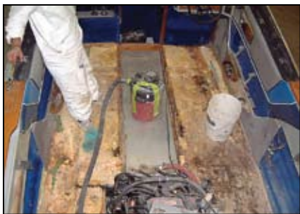
Removing the cockpit floor reveals the foam filled area below. Dark areas are wet.
