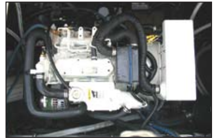
(top) Removing the old, rusty gen-set exposed an inadequate bonding system and resulted in a labor-intensive upgrade. (bottom) New 8kW Kohler fits the hold.
