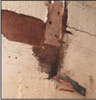
Digging out the wet deck from inside the cabin.
