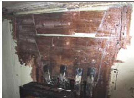
Ply layers epoxy glued back onto the bulkhead.
