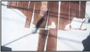
Plywood pieces removed from bulkhead and numbered.
