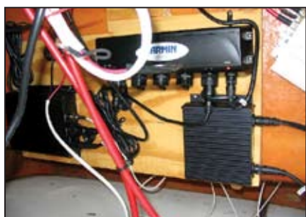
(top) Flying bridge with updated electronics. Chart plotter mounts on Navpod. (bottom) Network components mount underneath the bridge helm.
