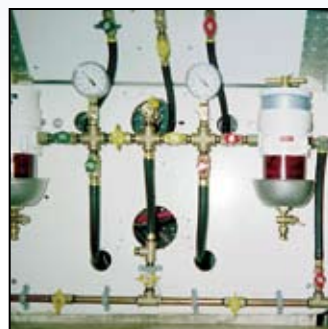
Amended fuel system incorporates ball valves, liquid-damped Racor pressure vacuum gauges and valves at the bottom of filter bowls for ease of servicing.
