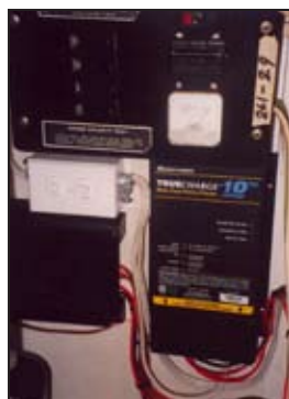
Electrical upgrades included a TrueCharge battery charger, AC electrical panel and a stereo amplifier (shown on the bottom left in the photo).
