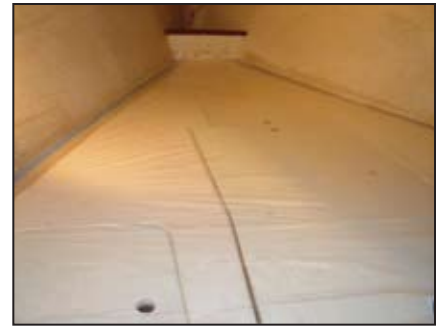
Patterning for a V-berth platform has masking tape under basting tape on the sides; pattern material in place and roughly trimmed.
