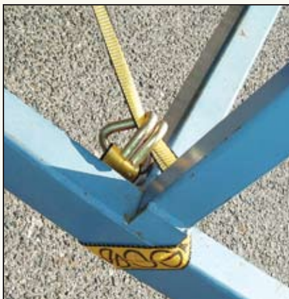
(top) Conventional welded eye for tie-down straps. (bottom) Ad-hoc tie-down strap attachment is just as secure as a welded eye but isn't as tidy.
