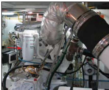
(top) Fuel from the tank passes first through a combined water separator and fuel filter, in this case, a duplex setup. (bottom) The engine manufacturers provide a secondary, spin-on type fuel filter mounted on the engine before the injector pump.
