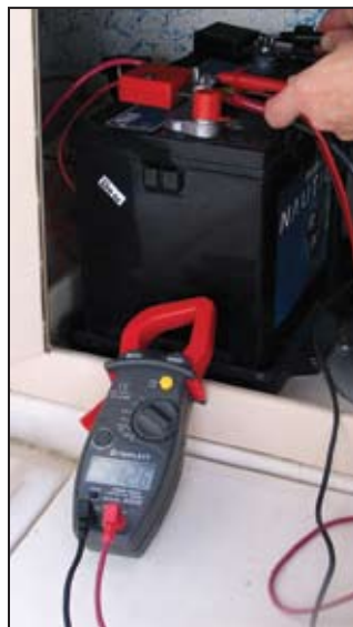
Measuring battery voltage with a digital clamp-on meter.
