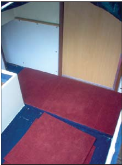
Dry-fitting the carpet tiles.
