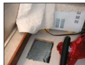
(across) Countertop cutout for larger air intake grill. (middle) Large cutout in front seat bulkhead for the return air grill. (bottom) Cut out in the countertop for one of two supply ducts with the other one installed in the forward cabin.
