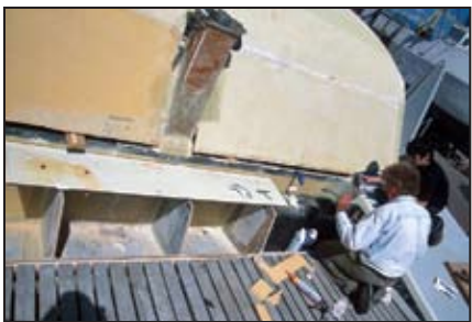
New fuel tank being installed in locker.
