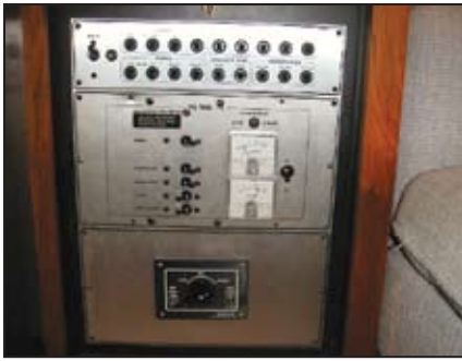
Combined DC and AC power systems' electrical panel.
