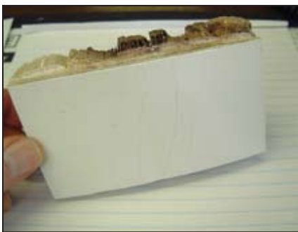
(top) The underside of a deck cutout. Note how the grain in this wet and deteriorated 3/4" (19mm) balsa core sample has opened up. Perhaps ruptured by frost? (middle) An inverted side view (cross section) of the same sample. Note the outer deck laminate is still well bonded and the area of worst deterioration is quite localized. A definite moisture hot spot. (bottom) A view of the outer skin and gelcoat of the same sample. Note the hairline cracks following the area of highest moisture in an otherwise "unstressed" part of the deck. Could this be a sign of stress from frost heave? Lab tests say no. Others say yes.
