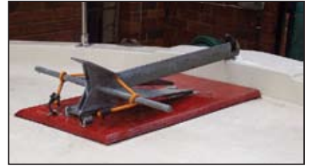
(top four photos) Before: Removing the hunk of anchor roller took some persuasion. (bottom photo) After: Anchor now mounts on a nicely varnished pad.
