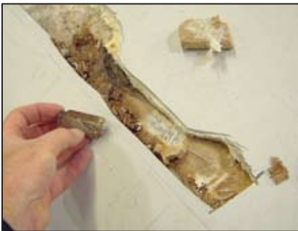
Digging out wet, rotten core, mostly from negligence rather than death by purely natural causes.
