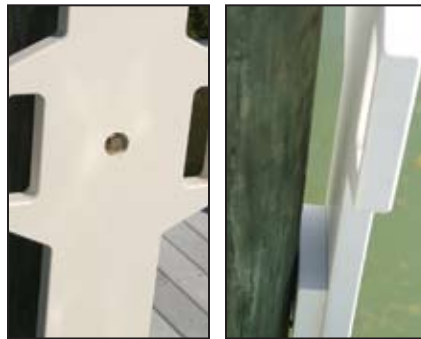
(left) Countersink your bolts so they don't scratch your gelcoat. (right) Details of backing block (standoff).
