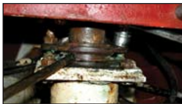
Detail of stuffing box shows (left) the screwdriver holding up the compression ring and (right) the socket over one of the tightening bolts.
