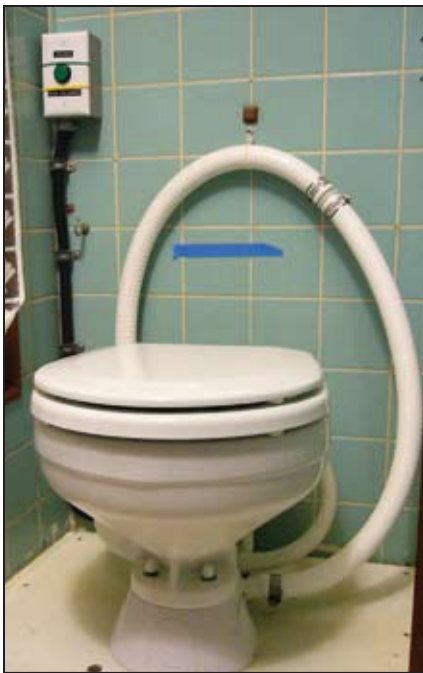
Cranky marine toilets are the bane of most boat owner's existence and are not as easily serviced as their household brethren.
