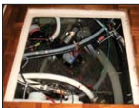
(top) Below-the-waterline thru-hull connects to a ball valve, though a seacock is the preferred installation. (bottom) Same fitting visible in right foreground as well as the maze of ducting, hoses and pumps.
