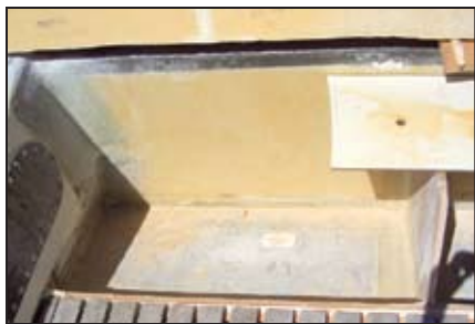
Lockers under construction. (top) The vacuum bagged panels have been taped to the existing cabin structure and some fairing compound has been applied to the seam. (bottom) New locker panels and partitions fiberglassed in place.
