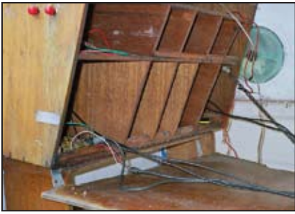
Original fusebox made of scrap wood.
