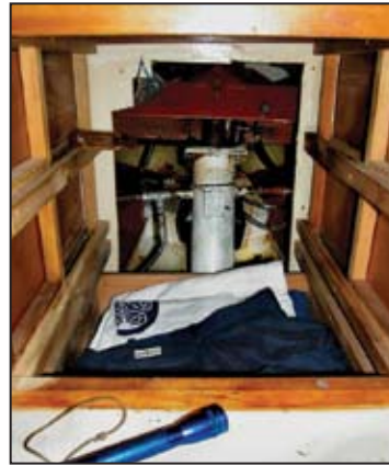
View of the rudder trunk and stuffing box as seen through the drawer space under the bunk.
