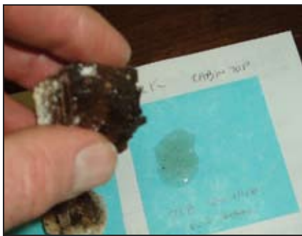
A fully saturated, rotted core sample. Note the pool of water left behind on the blue paper.
