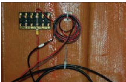
Wiring neatly placed inside locker behind the 12-volt receiver.
