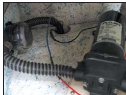
Pump reinstalled. Note heatshrink tubing over wiring connectors used to prevent corrosion and electrical shorts.
