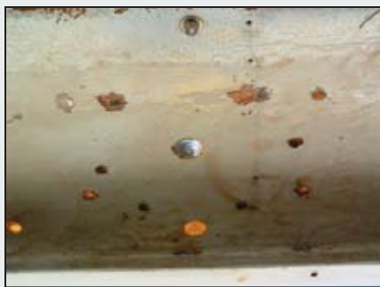
Fiberglass mat epoxied to the underside of the arch sealed the holes and provided additional reinforcement.
