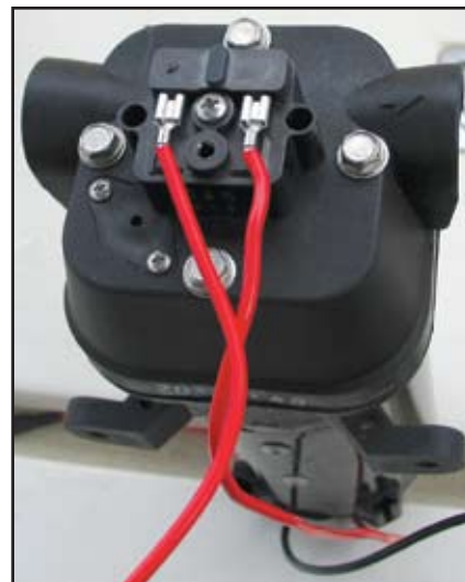
New upper housing assembly and pressure switch installed on pump.
