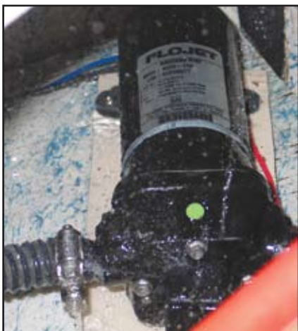
(top) Running plumbing anti-freeze through this washdown pump would have prevented the upper housing and switch from freezing and cracking, a condition that wasn't evident until the first use the following spring (bottom).
