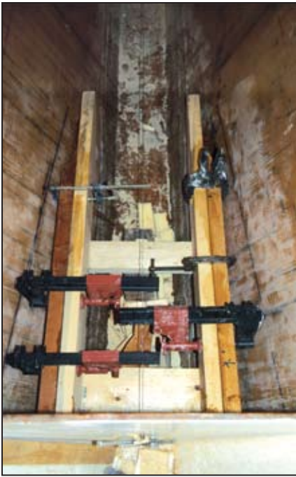
Engine beds glued together and clamped in position while the epoxy putty sets.
