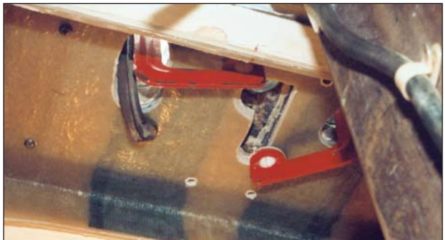
After a dry run to be sure of a good fit, the underside of the deck was ground clean and resin-coated to seal the plywood. A filler of polyester resin, two-parts microballoons, four-parts milled fiber, one-part Aerosil to the consistency of thick peanut butter and catalyzed at 2% relative to resin content, bonded the box to the deck.
