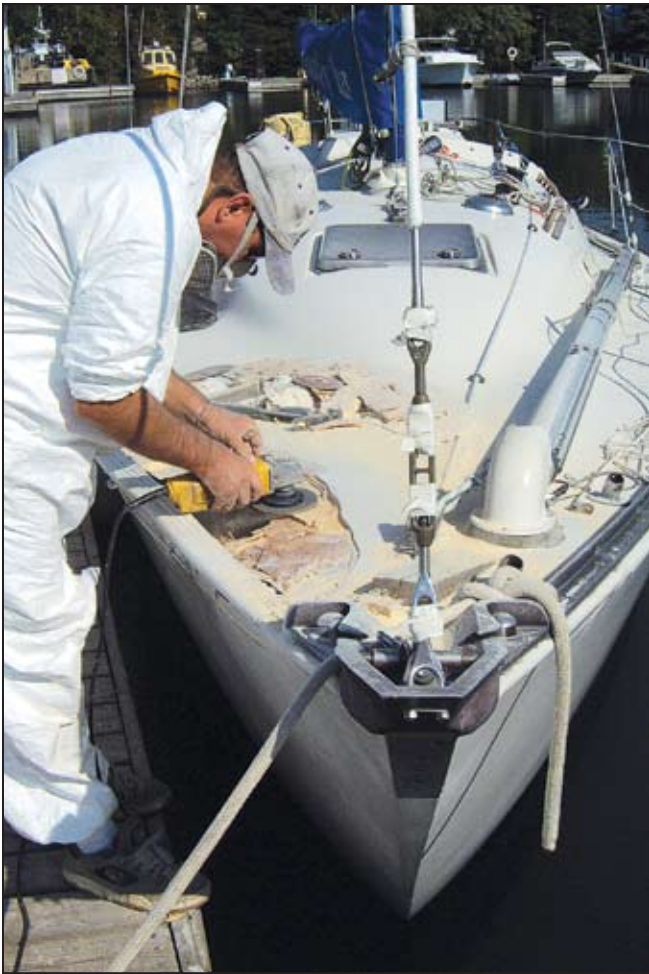
Unless you already have experience with major glass repairs don't jump in the deep end and try to replace a section of damaged core.
