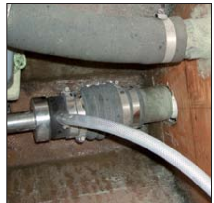
Shaft seal with vent hose and exhaust hose outlet, which has to pass through a watertight bulkhead so the connection is made through a fiberglass pipe glassed to the bulkhead.
