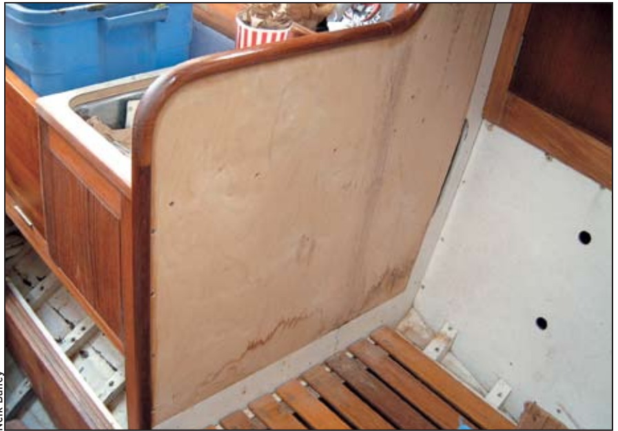
Removal of coating to bare plywood reveals water stains at the bottom.
