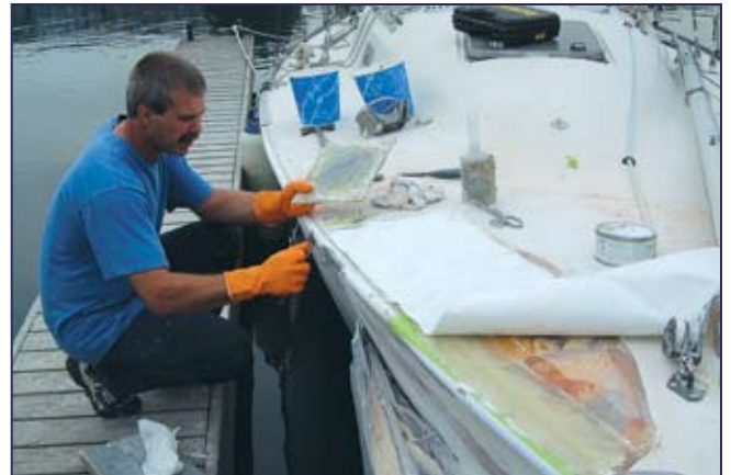
If you don't have the experience you are better off to leave major collision and storm damage repairs to a pro. The results must be "like new" otherwise it's a wasted effort.
