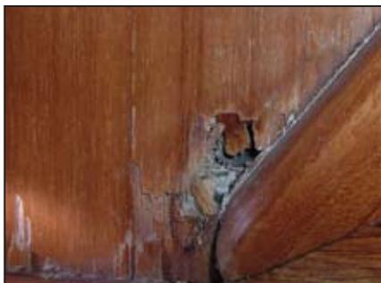
“Look behind the drapes.” This leak damage is typical of water finding its way in through window frames. The problem is most often seen in older Far Eastern built trawlers. Interior symptoms are easy to spot but the leaks often find paths between the outer fiberglass skin of the cabinsides and do serious damage to the laminate structure.
