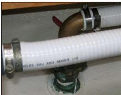
Hose connections are double clamped. Note proper orientation of clamp screws.
