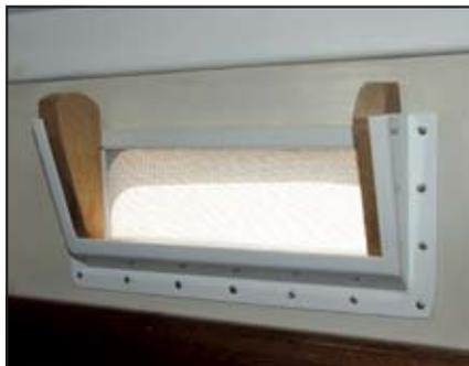
The screen fits within the port's frame, held in place against the interior surface of the cabin by wooden wedges.
