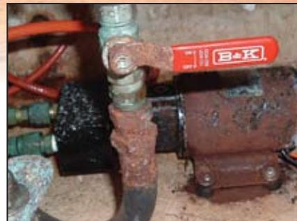
Everything still works but for how long? These fittings and the pump should be cleaned of rust and treated with a corrosion inhibiting formula to extend the life of all affected parts. A drier operating environment may not be possible but more corrosion-resistant materials should be considered for use here.
