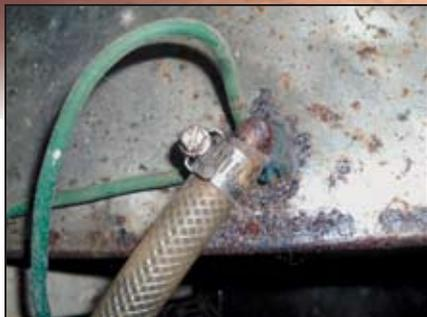
The bonding system connections had corroded to the extent that merely touching them separated their connections. The bonding system was there but, with only one broken connection, it was useless.
