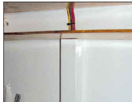
A simple white channel covers wires on the galley bulkhead.
