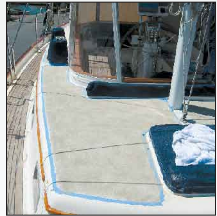
The medium, in this case 20-grit silica, was applied liberally to the first coat of paint. One layer of the regular tape was pulled after this application. The more medium that is applied, the better the chances of it being consistent but excess sand does get everywhere.
