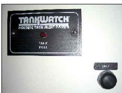
(top) Underside view of switch looking up inside the cabinet. (bottom) Switch on outside of cabinet. The "Head" sticker is a standard fuse panel label and cost $.50 at a marine store.
