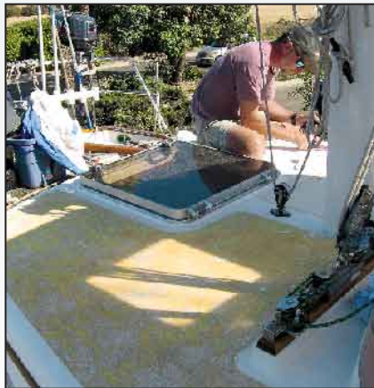
The starboard side with the non-skid removed, just prior to sanding. The yellow epoxy was markedly different from the white underneath on the port side.
