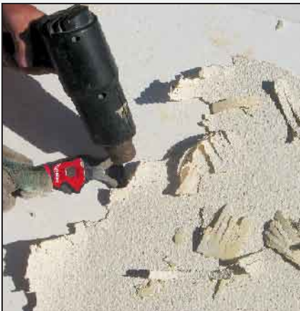
On the port side, where there were fewer cracks and no evidence of a previous repair, the removal was tough going, requiring multiple scrapers, a heat gun and lots of elbow grease.
