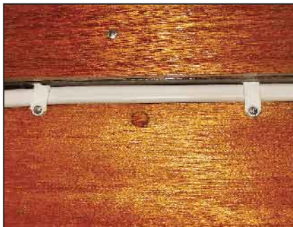
Wire clamped into a recessed area of the wheelhouse.
