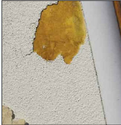
On the starboard side, which was apparently repaired once before with an epoxy base, the non-skid came off easily in large chunks.
