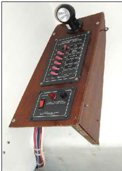
Neatly bundled wires exit the electrical panel.
