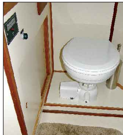
The finished installation. Note switch on left side of photo.
