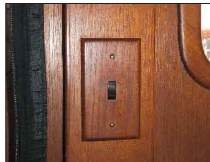
The light switch cover is stained to match bulkhead.
