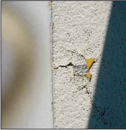
The first signs of non-skid failure on the cabin top appeared as bubbled areas, which cracked and ran in extended veins in all directions.
