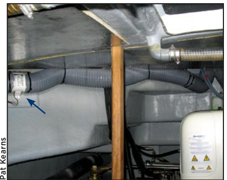
A system of corrugated vinyl hoses distributes the fresh air drawn into and blown out of the engine space by the inline blower motors (as shown by the arrow). The engine air intakes take care of pulling in the cooler air needed for efficient engine combustion.
