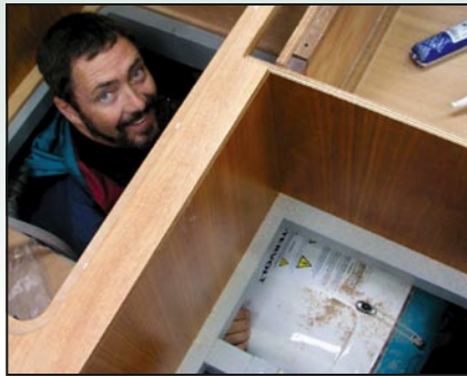
Mastervolt Whisper 3.5 kW fits snugly under the raised salon floor of this 40' (12.1m) sailboat. Service access is through a dinette seat locker.
