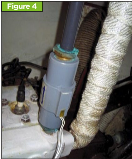
(above) Aqualarm water sensor mounts to the exhaust water jacket on the manifold. Covered stainless-steel riser pipe connects to the exhaust manifold. (right) View of Aqualarm, riser pipe and connections. Black exhaust hose leads aft to Vetus muffler in the lazarette.
