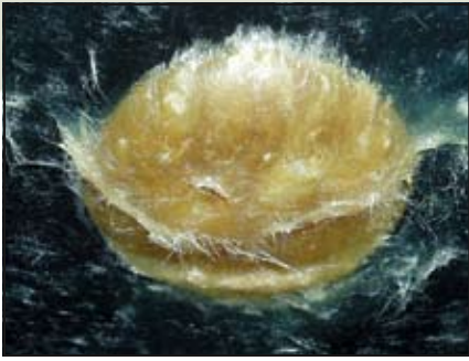
A solid glass and resin plug fills the void between the skins and bulges out of the repair access hole.
