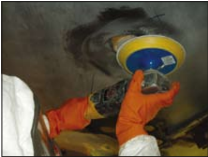
A 1,500-rpm sander with a flex pad and 80 grit disc is used to flatten and recess the bulging plug.
