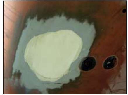
(top) The cured fairing putty is block-sanded flush with the hull with 80-grit paper to (bottom) yield a smooth, level surface for the patch that is paint ready.
