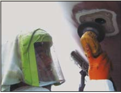
Use a grinder and a 36-grit disc to carve a bevel into the hull laminate around the hole.
