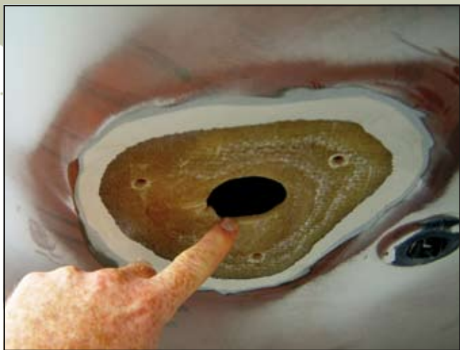
After prep grinding, note the laminate layers exposed.
