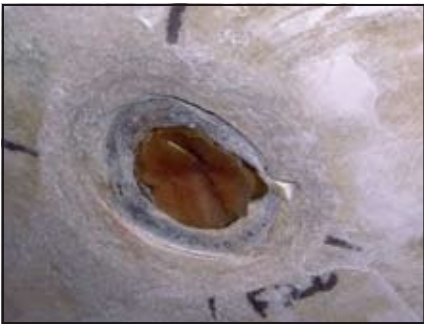
The beginnings of a beveled scarf face around a thru-hull to prep it for a glass cap. This one needs to be a bit larger to achieve a 12:1 ratio.
