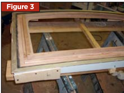
The combination lip and coaming placement was done to maximize window size.
