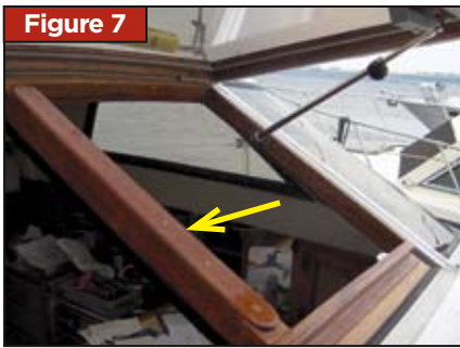
Figure 7 Vertical support bar was added after deflection tests suggest a potential weakness.
