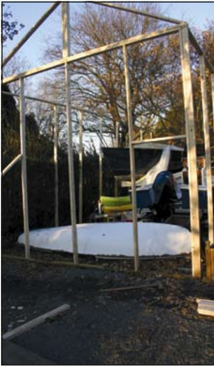
Shrinkwrap shed under construction.
