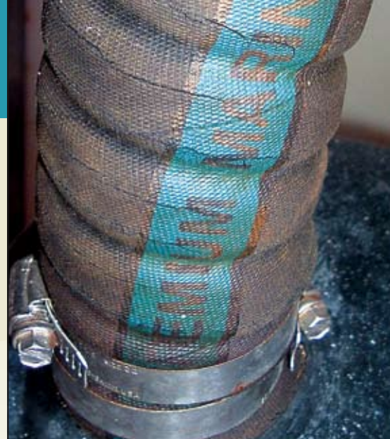
A cracked hose shows that even "certified" hose can fail when it exceeds its service life.
