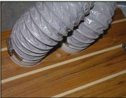
(top) Mounting board cut and drilled for inverter/charger and vent grilles. (middle) Mass Combi 12/2000-100 and 3" (76mm) vent grilles fitted to backboard that is secured to a floor bearer. (bottom) Vent ducting attached to grilles.
