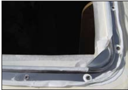
Sealant squeezes out the edges and screw heads as fasteners are tightened.
