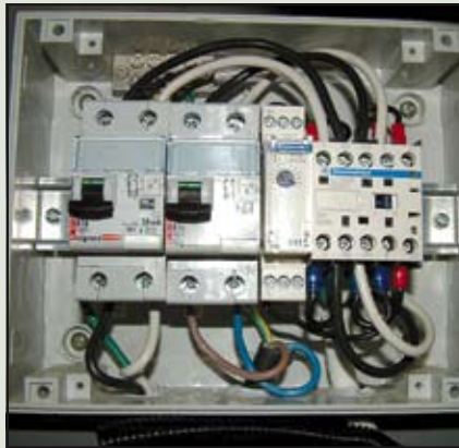
Removal of the front protective panel on Mass Combi provides access to AC terminal connections. The "short break" output is the right terminal block.
