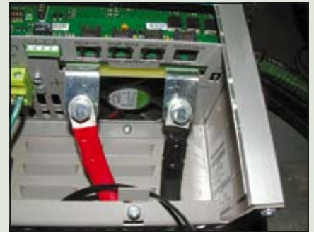
Positive and negative battery cables connected to inverter/charger.
