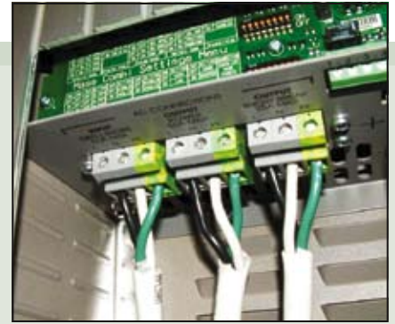
Removal of the front protective panel on Mass Combi provides access to AC terminal connections. The "short break" output is the right terminal block.
