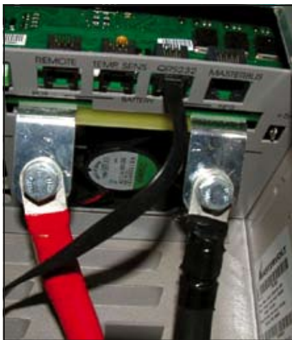
Black wire connects the remote control panel via a telephone jack connection.
