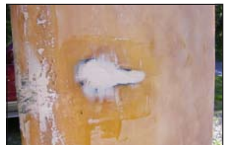
While the epoxy was still tacky, gouges and dings were filled with a mixture of epoxy, colloidal silica and fairing compound.
