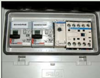
(top) Generator and shorepower input cables connect to terminals in the Masterswitch. (middle) Auto changeover switch and connections (visible on the right side of the switch box). (bottom) Protective see-through cover shields switch box wiring.
