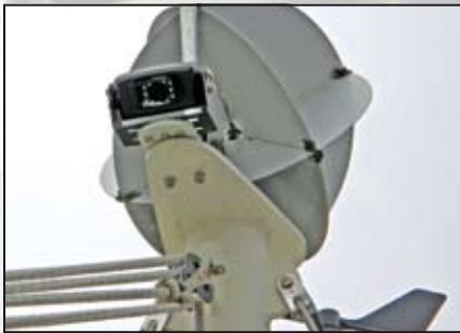
Camera bracket bolts to the trailing edge of a small aluminum extension plate that fastens to the existing tower plate.
