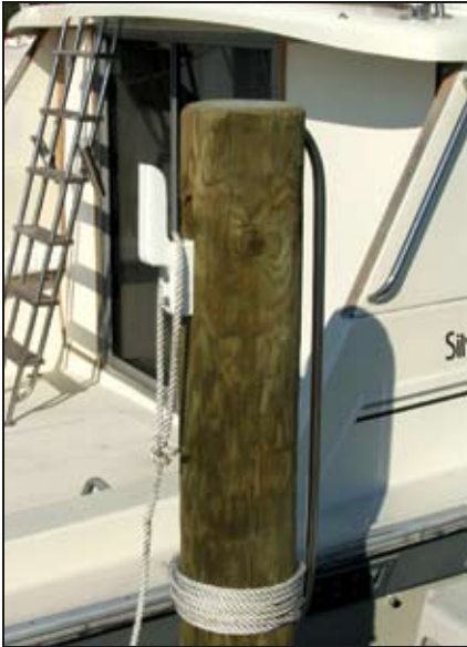
Sturdy hooks attach to any piling to keep lines dry and accessible.
