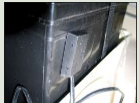
Temperature sensor connects to a battery on the house bank and signals an alarm should the battery overheat when charging.
