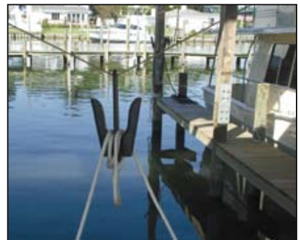
(top and bottom) A bracket hanging from the roof of a covered boathouse makes it easy to drop or pick up bow lines.
