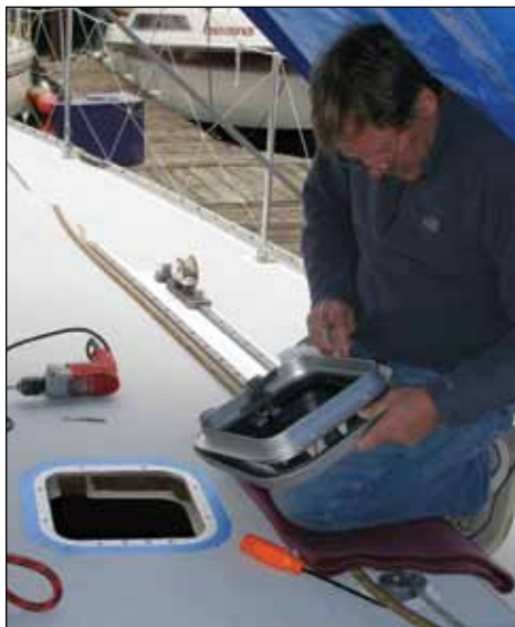
David completes a final cleaning and dry fit before sealing and affixing the new hatch.
