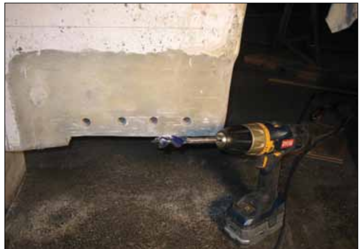
Oversized holes were drilled, then filled with epoxy. Later, the holes for the skeg bolts would be drilled into this epoxy, leaving the interior of the keel completely sealed.
