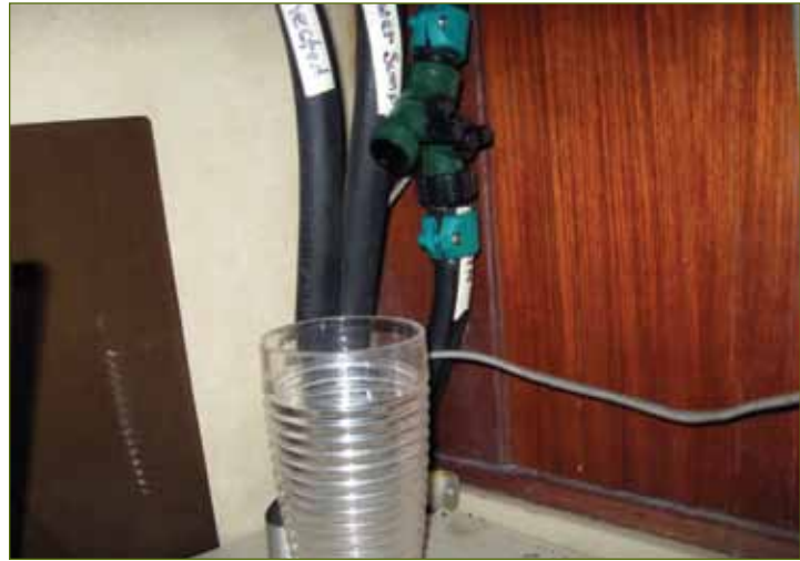
The system allows the author to stop all storm water, flow it through to the through-hull, or divert it to use elsewhere on the boat with a hose.
