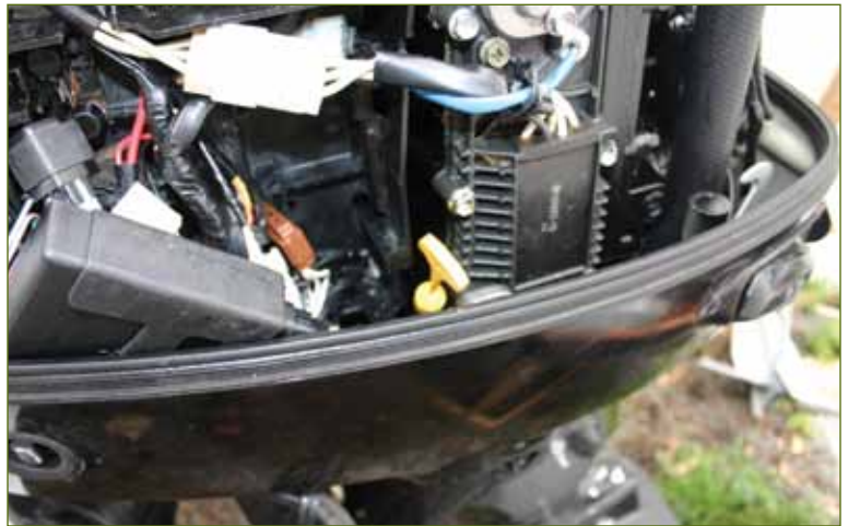
Using needle-nose pliers assisted with some of the connections, but accessing some screws proved to be difficult because of the tight space.
