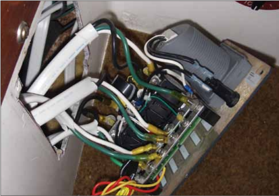
ABOVE: Wiring the main distribution panel.
