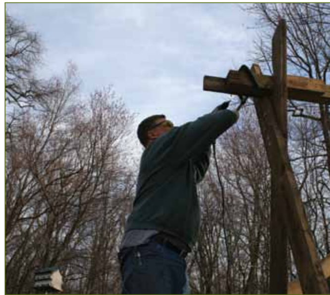
Make sure all the wood for your gantry is in good condition and use clamps to hold the pieces while you prepare to through-bolt the sections together.
