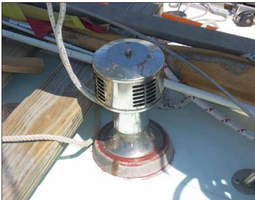
The completed "Charlie Noble," or ship's chimney. Note the red heat-resistant sealant between the teak and the stainless collar, as well as between the teak and the deck.
