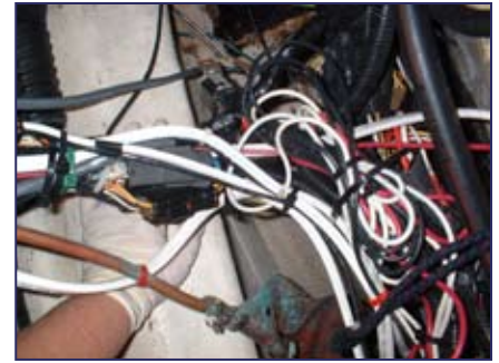
This is an electrical stew recipe from a shade tree electrician: a little AC; a little DC; some electronic cables; and a fuel hose.
