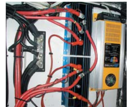
Smart chargers and battery isolation diodes allow the alternators to charge multiple batteries.
