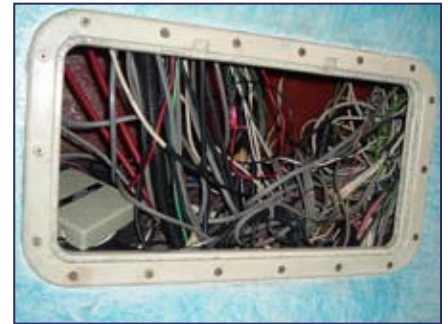
Troubleshooting this wiring spaghetti is an electrical nightmare. This is a candidate for a "do over."
