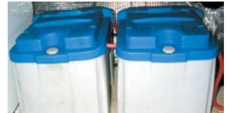
Screw-down covers that hold these batteries securely in place, even in rough seas. They also cover the terminals so nothing metallic can short-circuit them.
