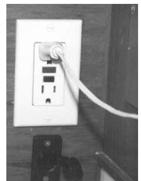
AC outlet receptacle with GFCI, reset and test buttons to protect the user from line-to-ground electrical shock hazards.
