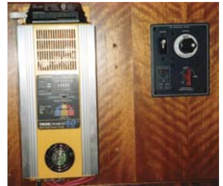
Two three-way battery switches are removed (top) and replaced by a DC Parallel Circuit Battery Switch (bottom). TRUEcharge 40+ multi-stage battery charger at 40-amp output is one of the biggest available.
