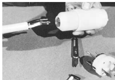
When a bad shorepower connection develops, splice a new plug or connector onto the cordset.
