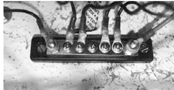
Dedicated terminal block for negative wires.
