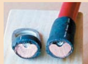
Example of what a good crimp looks like after the hammer blows. Note how the strands of the wire and the walls of the lug appear as solid copper.
