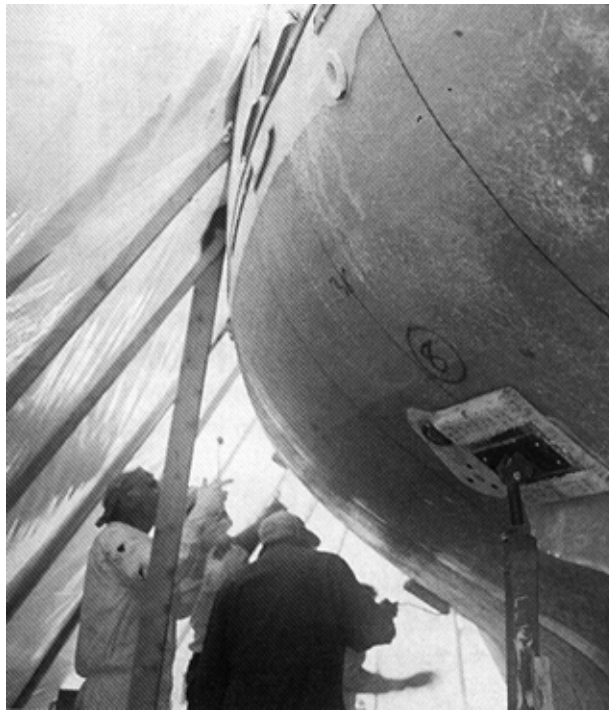
The hull was divided into sections and labeled with a waterproof marker in preparation for applying the new laminate. The lighter area below the waterline is the Airex core which remained intact.
