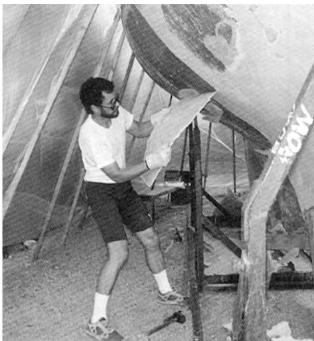
The outer layer of fiberglass peeled off the hull in huge sheets — like peeling a banana!
