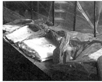
Mat and roving were precut and labeled so they could be applied without stopping.
