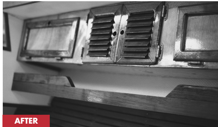
A more functional cupboard with horizontal and louvered doors and a lower shelf with fiddle.
