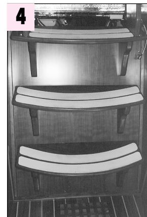
Adhesive-backed non-skid tape applied to companionway steps.
