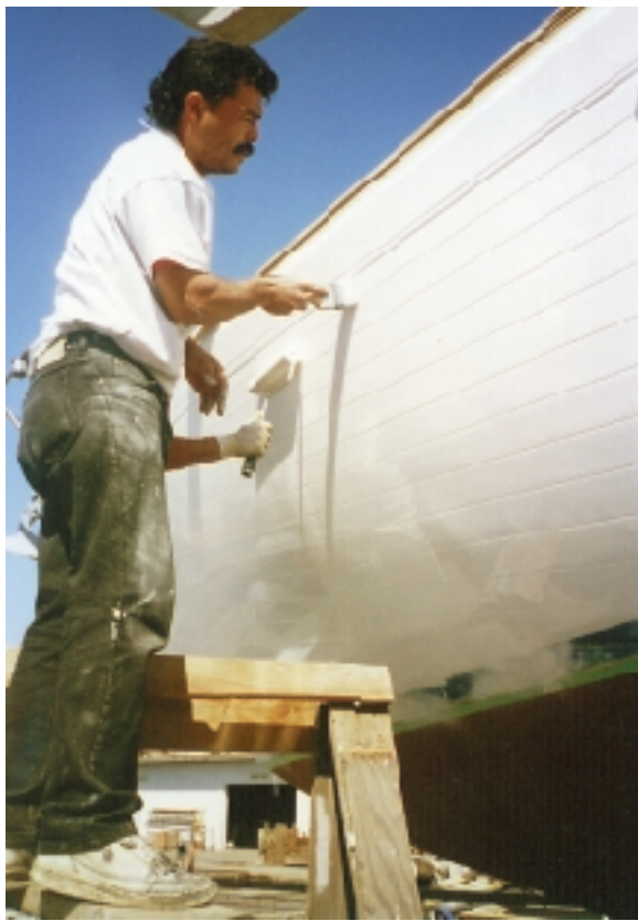
Rolling and tipping: The paint is first applied vertically with a foam roller then “tipped” by brushing in the opposite direction. The painters in this photo are not wearing the proper safety attire.
