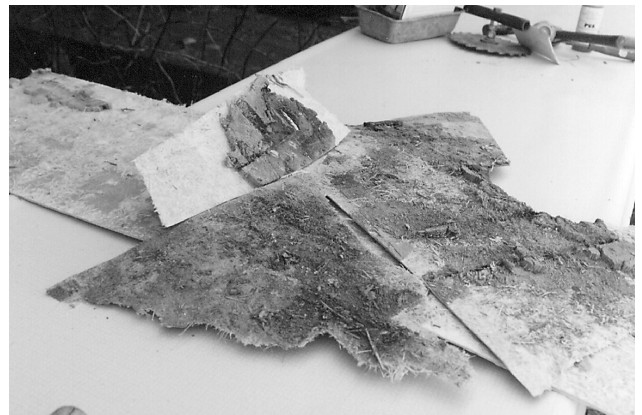
Strips of the outer deck laminate showing the rotted core.
