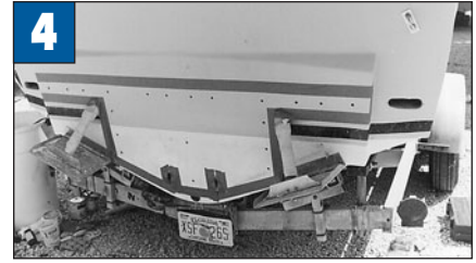
4 Transom prepped with wide masking tape, tab cylinders and thru-hulls covered, and bolt holes drilled.
