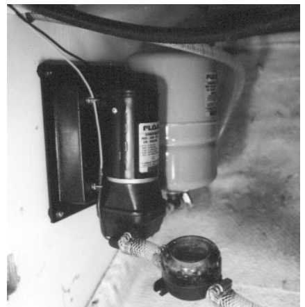
FLOJET model 2840 Water Pressure System mounted on an engine room bulkhead. Note strainer in foreground.
