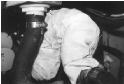
Exhaust riser wrapped with insulation secured with stainless-steel wire.
