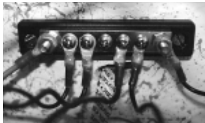
Panel rewired with a negative bus bar for attaching negatives from gauges. Negative lead from ignition control module is shown on the left, negative lead to "GND" on tach is on the right.
