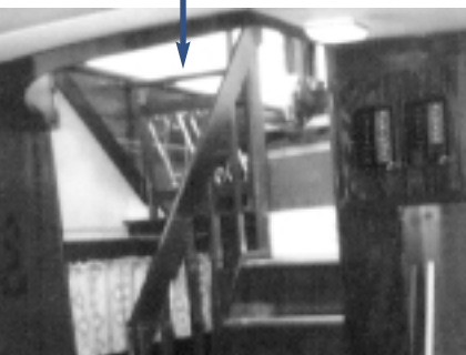
View from below with newly installed electrical cabinet, breaker panels and wiring chute. (top) Headliner constructed of fir plywood, stained and varnished, completes entranceway.
