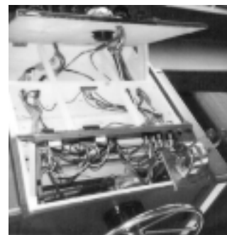
(right) Top panel opens for easy access to wiring. Note neat and orderly wiring job.
