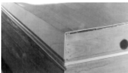
Plywood is dry fitted and marked for realignment during permanent installation.
