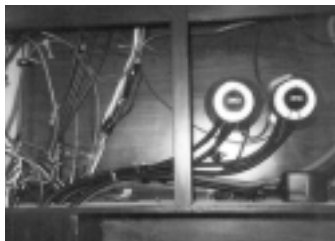
(right) Electrical cabinet and 12-volt breaker panels for house loads. (top) Wiring and dual battery switches inside cabinet.
