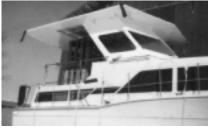
Aluminum hardtop temporarily supported on deck.
