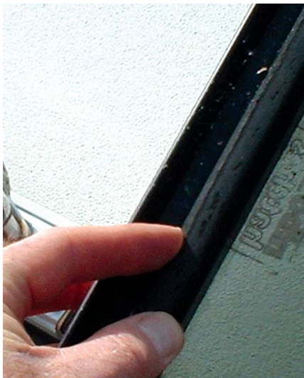
Close-up of gasket on edge of hatch lid with frame.
