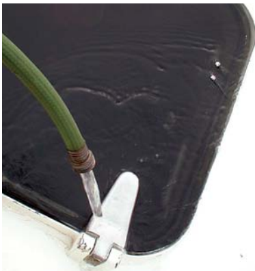
Leak testing with hose.
