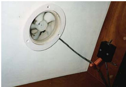
Underside of aft hatch shows mounting of two-speed switch.
