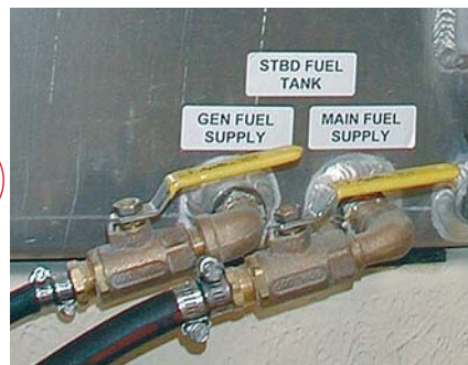
Separate fuel pickups for each of the two main engines, gen-set and cabin heater. Bushings made of 500 series stainless steel provide a galvanic barrier between the copper-based alloy fittings and the aluminum tank.
