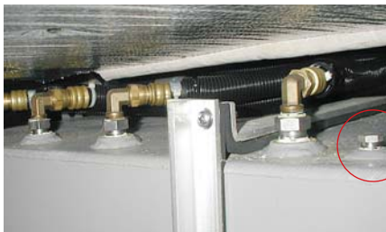
Separate fuel outlets and valves for the gen-set and the main engine. Note the shutoff valve at the bottom of the sight gauge.
