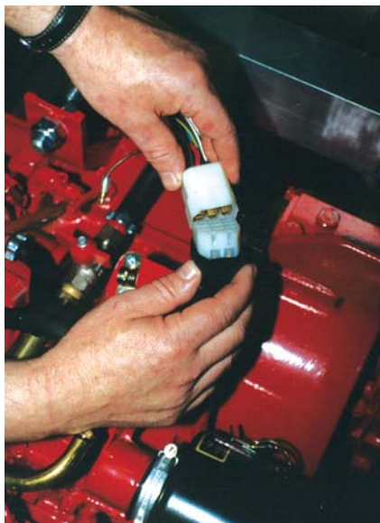
Inspect fuse blocks for corrosion.
