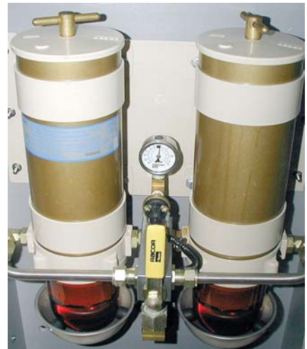
Dual head (duplex) filter arrays allow one filter to be serviced while continuing to operate through the other. Note the sender/switch teed into the vacuum gauge. It's wired to an indicator on the bridge.
