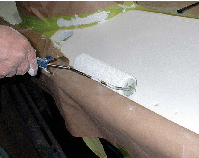
FIGURE 6 Stucco-style non-skid applied with paint roller.
