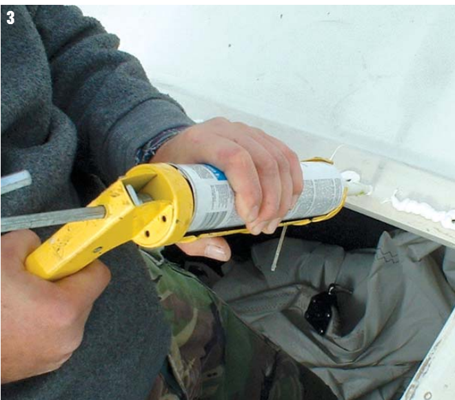
Steps to resealing a hatch frame: 1 Break the seal by gently driving a putty knife between the hatch base and deck. 2 After hatch base is removed, scrape off the old sealant. 3 Apply new sealant, being careful to plaster each fastener hole well.
