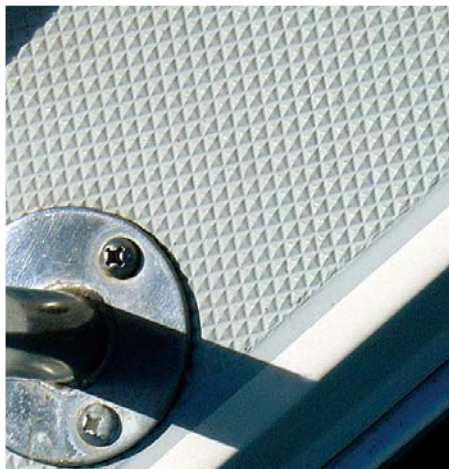
FIGURE 1 Close up of diamond repeating pattern non-skid.
