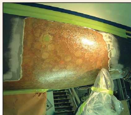
Minor osmosis is no immediate threat but shows hydrolysis is at work. Time for a barrier coat before things get worse.
