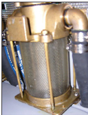
Check for crud in water intake strainer.
