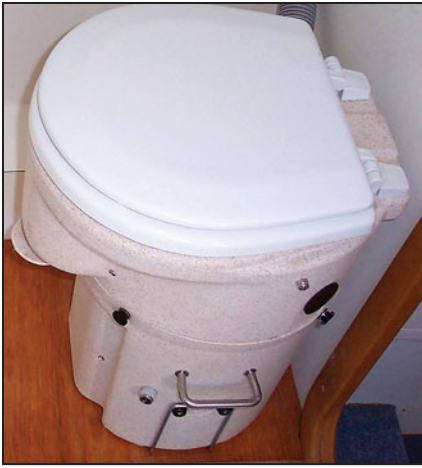
Air Head installed in hold-downs and ventilation hose attached. The liquid container is not in place.
