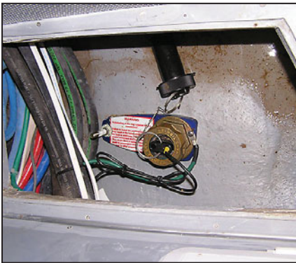
Lift floorboards and check for debris.
