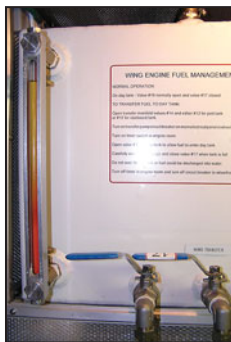
Well marked fuel tank.
