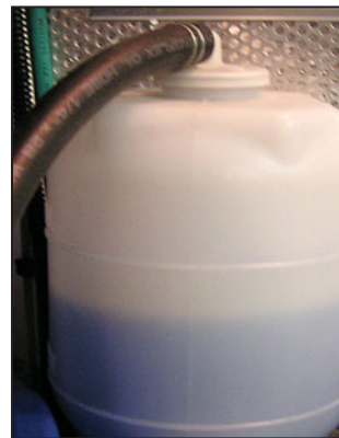
Check coolant level in overflow reservoir.
