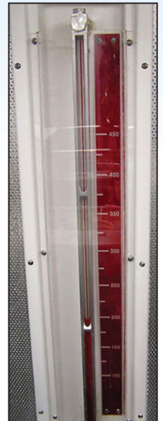
Sight Gauge Fuel Tank
