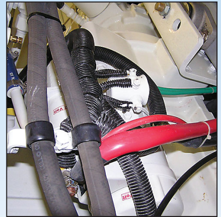
Look for chafe on hoses.
