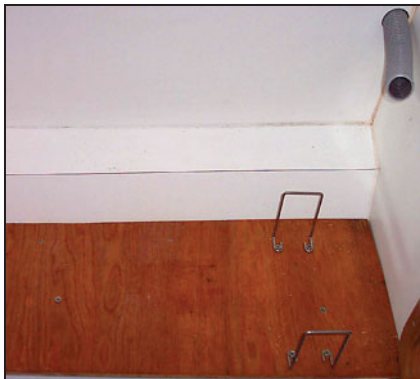
New head platform made of epoxy-coated plywood, with vent hose and Air Head hold-downs in position.
