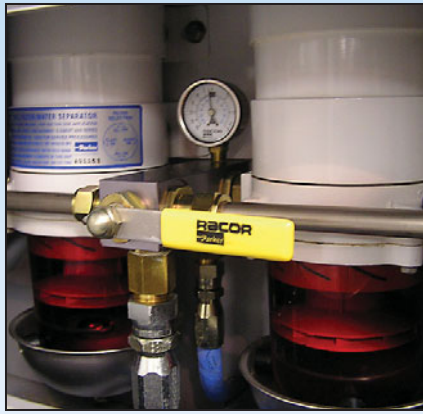
Every hour, check sight bowl for water in fuel filter/water separator.
