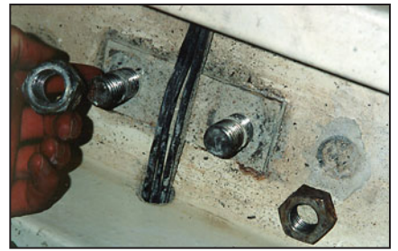
Typical top-end installation with backing plate and washer.
