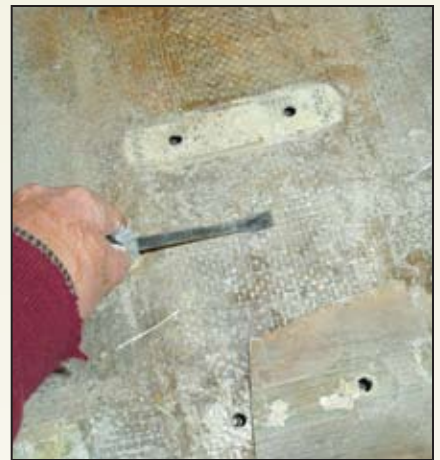
Not a pretty sight, keel bolt locations were delaminated and stained from water leaking through the laminate. Note the white resin-starved appearance of delaminated glass.
