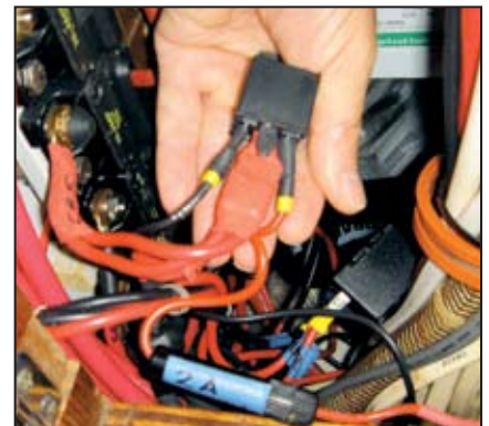
Isolating relay and clearly marked 2-amp inline fuse. Note use of heat-shrink tubing for corrosion protection.
