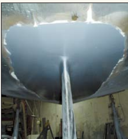
Exterior fairing done and repair epoxy primed.
