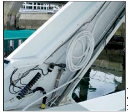
As a rule, it's not recommended to cut cables but coil them instead in neat bundles in a concealed area (inside the radar arch in this photo).
