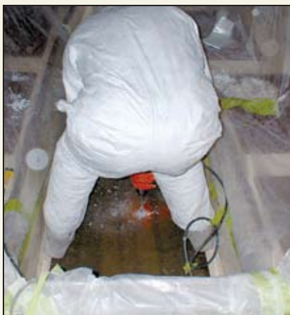
Drilling the keel bolts. Note the glow from the guide light outside the hull.
