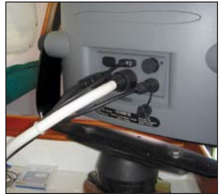
Aside from a new mounting plate, the new scanner was a simple bolt-on installation. Be sure cables are long enough to provide strain relief and a "service loop" so you can turn the equipment to examine the backside.
