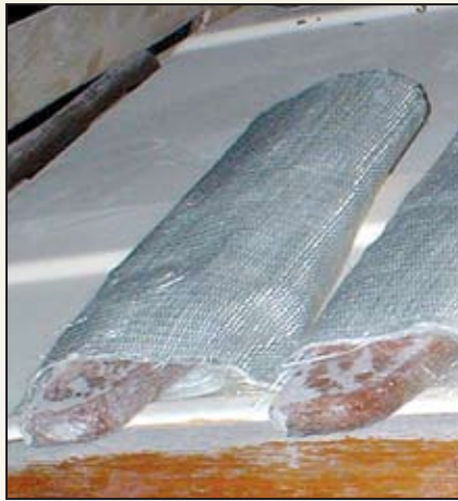
New floor beams with glass kits awaiting installation.
