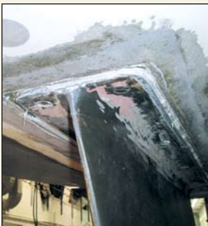
New external glass in place and the keel fitted; filling and fairing is pending.
