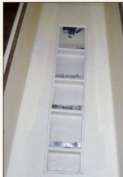
The completed job, painted with air-dry gelcoat and with the sub-floor glassed back in place.
