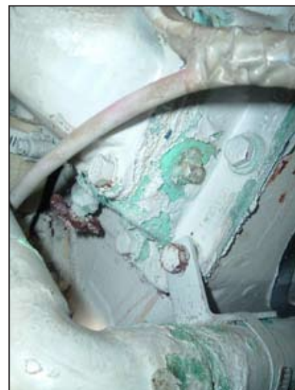
The "aerosol overhaul" of white paint didn't stand up to the corrosion activity beneath.
