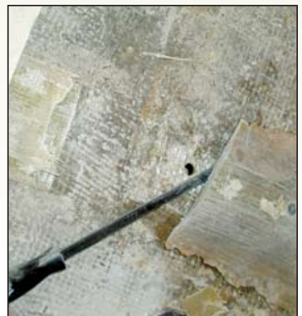
The hull layer attached to the Lyasil web is delaminated badly enough to be peeled back with hand tools.
