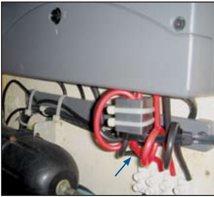
Loop power supply and negative cables through ferrites and secure with wire ties.
