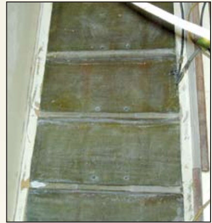
The new floor beams glassed in place.
