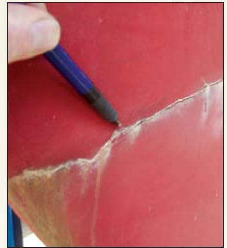
This sort of keel-hull joint crack looks bad but may indicate only that the keel bolts need tightened.
