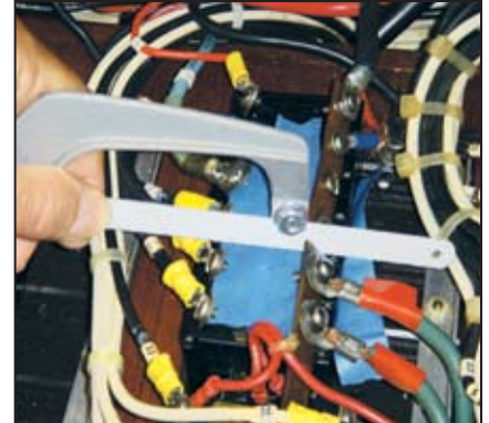
Cutting the circuit breaker bus bar. Strips of tape, adhesive side up, capture metal filings.
