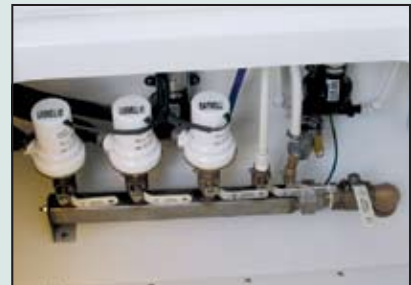
There's no mystery here as to which valve operates what pump and it's all nicely bundled in a compact, well-engineered manifold.
