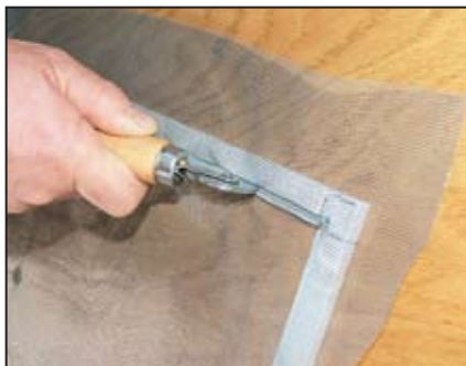
Use the spline tool to press spline in place.
