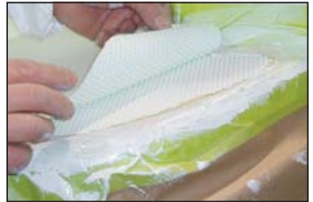
After the gelcoat has cured peel back the Flex-Mold to reveal the new non-skid. Note the rough edge overlapping onto the masking. This is trimmed off and sanded.
