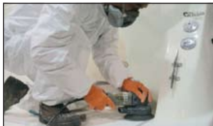
The existing non-skid in the repair area is removed by sanding with 40 to 80 grit dry paper.
