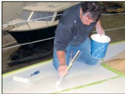
When repairing decks, select a resin compatible with your choice of finish coating.
