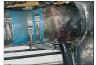
Exposed fibers found on the exterior of a FRP section of pipe dictate that the pipe be removed and examined carefully for symptoms of degrading laminate.
