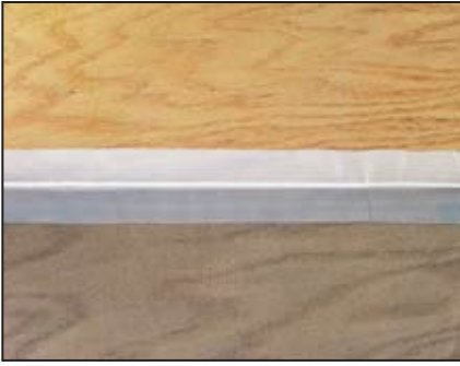
Place 3/16" (4.7mm) line and screening onto tape at the fold line.
