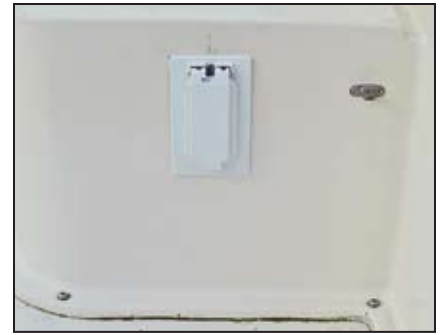
GFCI receptacle mounted on the flying bridge locker.
