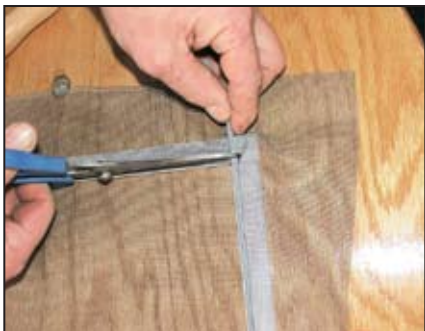
Cut the spline to fit flush; press in the cut end.
