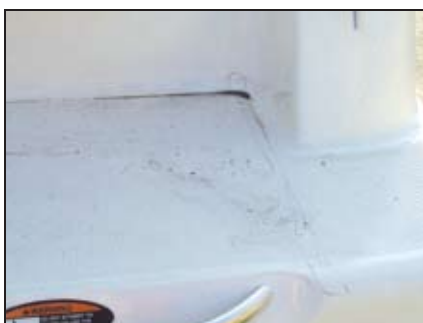
Without Gibco Flex-Mold, the cracks traversing this swim platform would be difficult to repair while preserving the original non-skid pattern.
