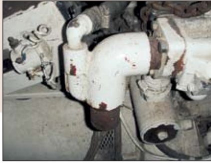
Seawater joins the exhaust at the exhaust elbow causing aggressive corrosion and clogging.
