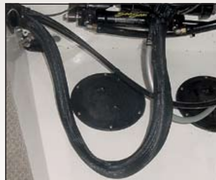
Protective sleeve contains the engine wiring harness.
