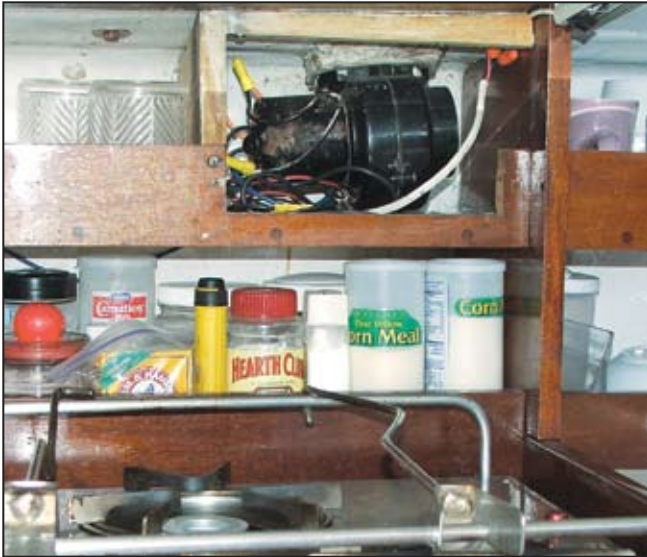
Blower installed in shelf area above stove. Metal screen filter covers the blower compartment.
