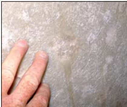
Exposed hydrolyzed laminate with weeping blisters requires more laminate removal.
