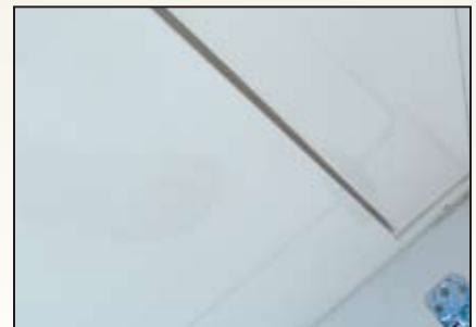
A mis-aligned bi-fold door leading into the cuddy cabin of an offshore fishing boat was the entry point of a persistent leak.
