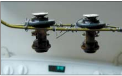
Thermostats out of the water showing fully open.
