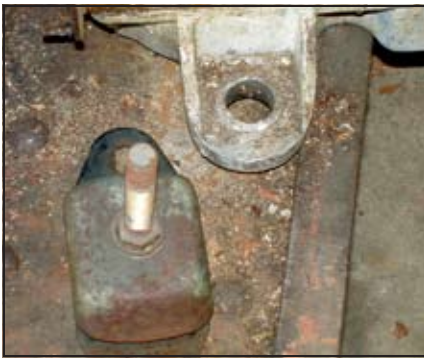
Incorrect bracket hole to mount post size creates movement in the system, resulting in vibration and possible component failures.
