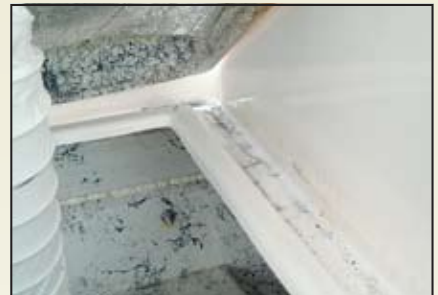
Hatch has shallow flanges in the cockpit sole molding and no drain. The boat was stored on a lift, slightly bow down so that rainwater flowed over the flanges and into the bilge. During a continuous rain, the water ingress overtook the bilge pump's ability to pump it out and everything became saturated, rusting and corroding the transmission, coupling, engine mounts, etc.
