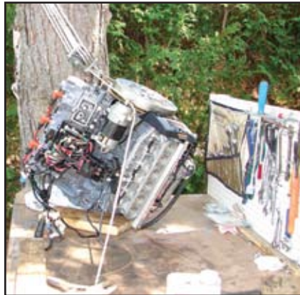
Getting the power head ready to lift.
