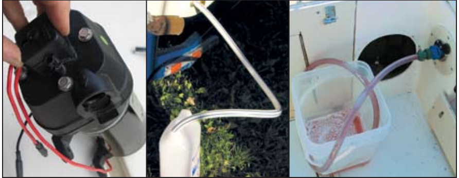
Residual water in the pump froze and cracked the housing and switch.
