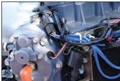
Wire connections running above port head.
