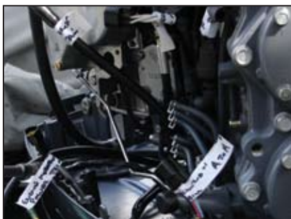
Labeled wiring for the engine mounted power trim.
