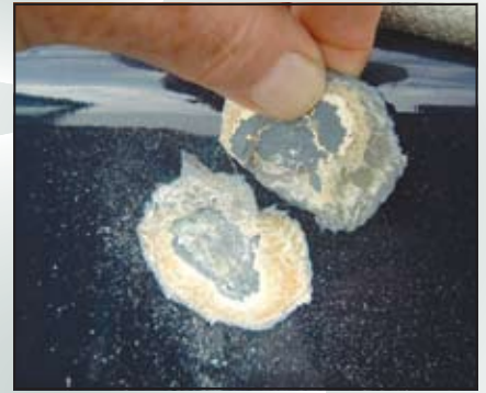
This topside blister in a custom fiberglass hull originated in original construction when glass was layed over paint primer.
