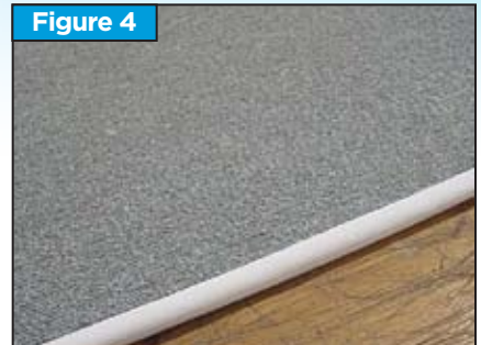
Finished carpet edge bound with a facing.
