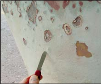
An ugly collection of blisters that is affecting only the keel fillers and bottom coatings.
