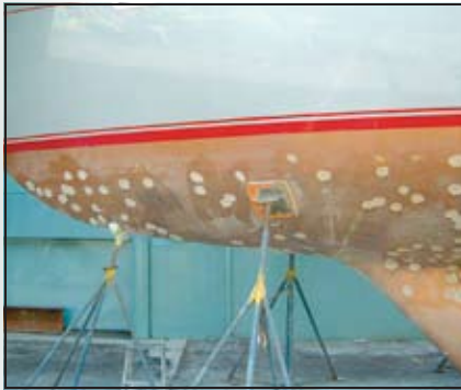
A blister spot repair underway. This example is near the outside limit of spot repair practicality.
