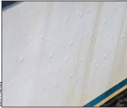
Fire-retardant resins used on this boat apparently caused blistering above the waterline.
