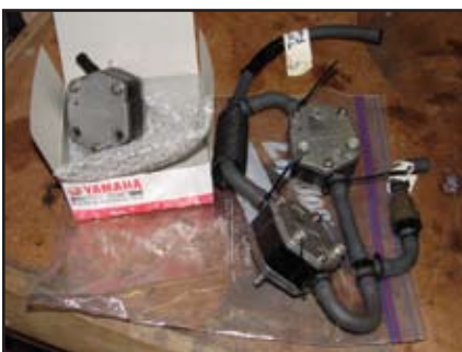
Installing two new fuel pumps. These pumps have a right and a wrong way to install them. Make sure the arrows are going in the right direction.
