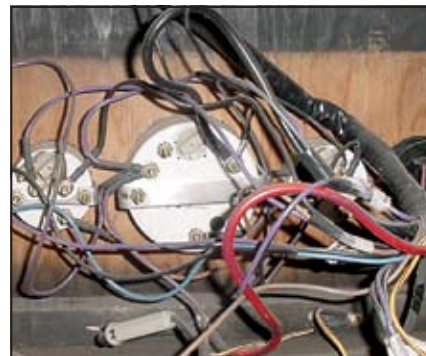
This wiring mess should be tied and secured to reduce the possibility of broken wires.
