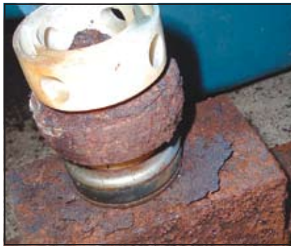
Badly rusted mount needs replacing.
