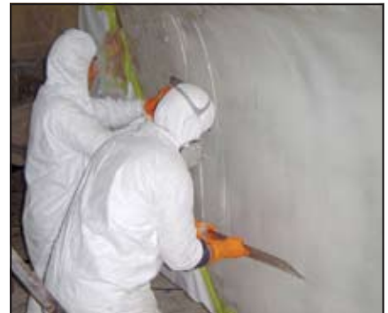
A fairing team at work pulling putty.
