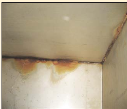
Corrosion along the weld lines created pinhole leaks in this freshwater tank.
