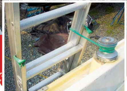
(top). The scene of the accident, a long way to fall. (inset) Bungee tied to a winch prevented the ladder from kicking completely out and dropping me to the ground.
