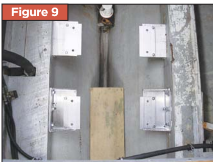
Ready for the new engine.
