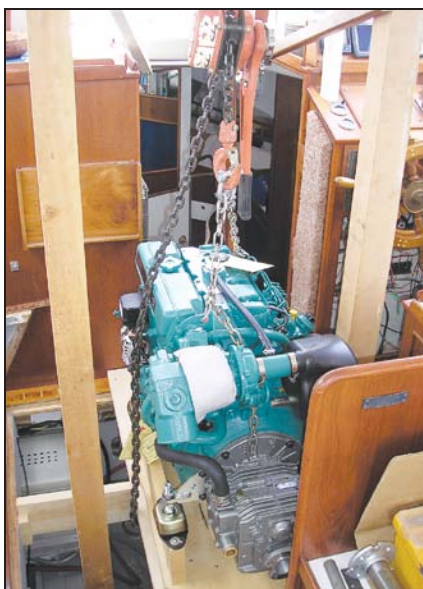
(top) Pulling the new engine into the cabin. (bottom) Lowering the new engine into place.
