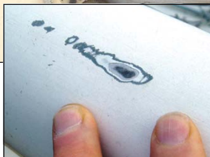
A close inspection of a chafed spot on the wishbone shows a good base with two layers of paint and primer. This will be the boom's third overcoat paint job.
