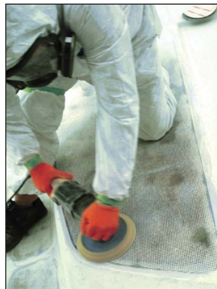
Removal of original non-skid pattern using a 1,500 rpm polisher fitted with a foam pad and 40-grit disc. Only use a sanding tool this aggressive to prep non-skid areas that will receive a textured finish. Note haz-mat gear worn by the technician — these are nasty materials!
