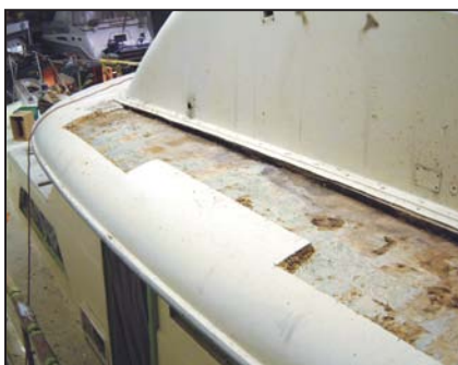
Major core repairs are a good reason to refinish a deck.
