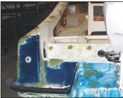
Underlying fiberglass problems, including minor gelcoat cracks, require repair prior to painting.
