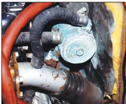
(top) Proper installation of a vented loop. (bottom) Vented loop not installed on engine.
