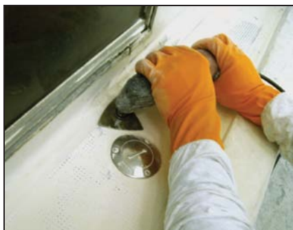
Most detail prep-sanding must still be done by hand. Tools like this Fein edge sander can help speed up the work.
