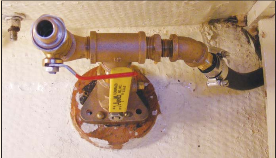
Final configuration of the new seacock/engine flush configuration with emergency hose and strainer. The hose will be lengthened.
