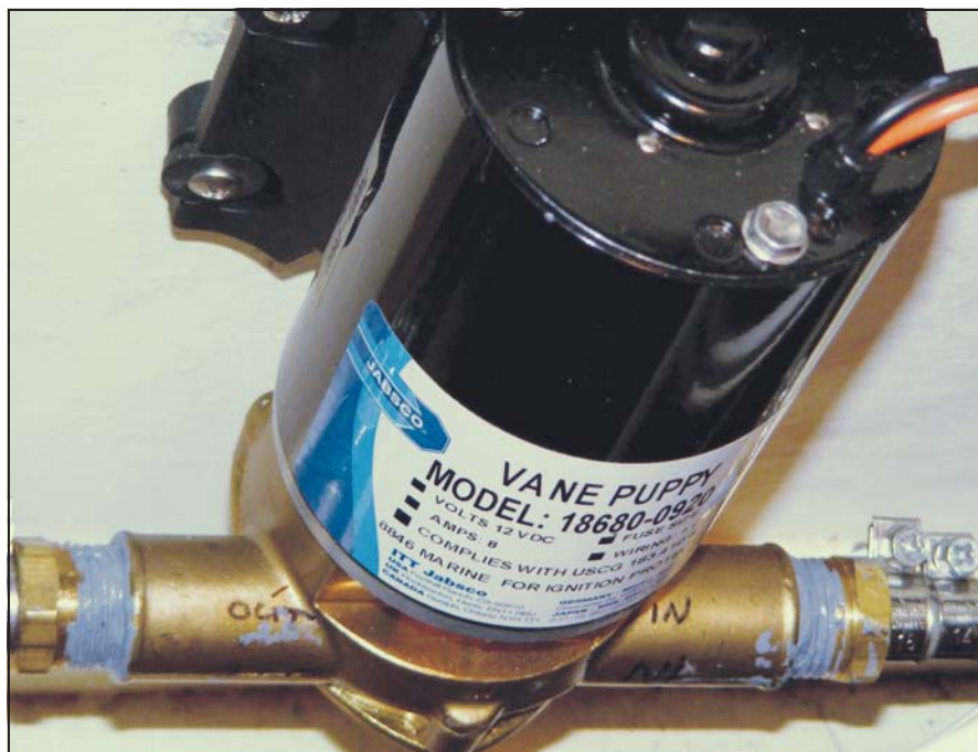
A stand-alone rotary vane pump is the best choice for supplying fuel to the stove.
