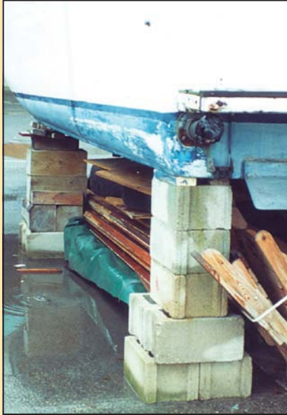
Bad: Never use cement blocks as they are prone to failure under boat loads.
