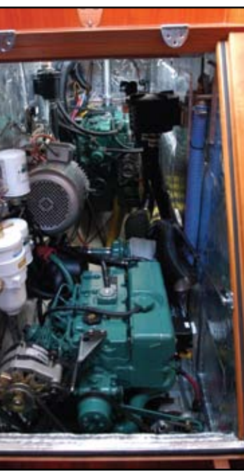
The author's engine room with a conventional diesel in the foreground and experimental parallel electric on the upper left with the electric propulsion generator in the background.
