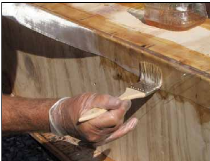
Fill and apply fiberglass to all seams on the exterior of the box.
