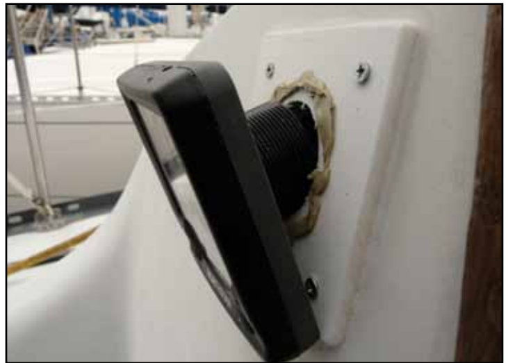
A piece of Starboard was used to hide the old holes and mount the new unit.
